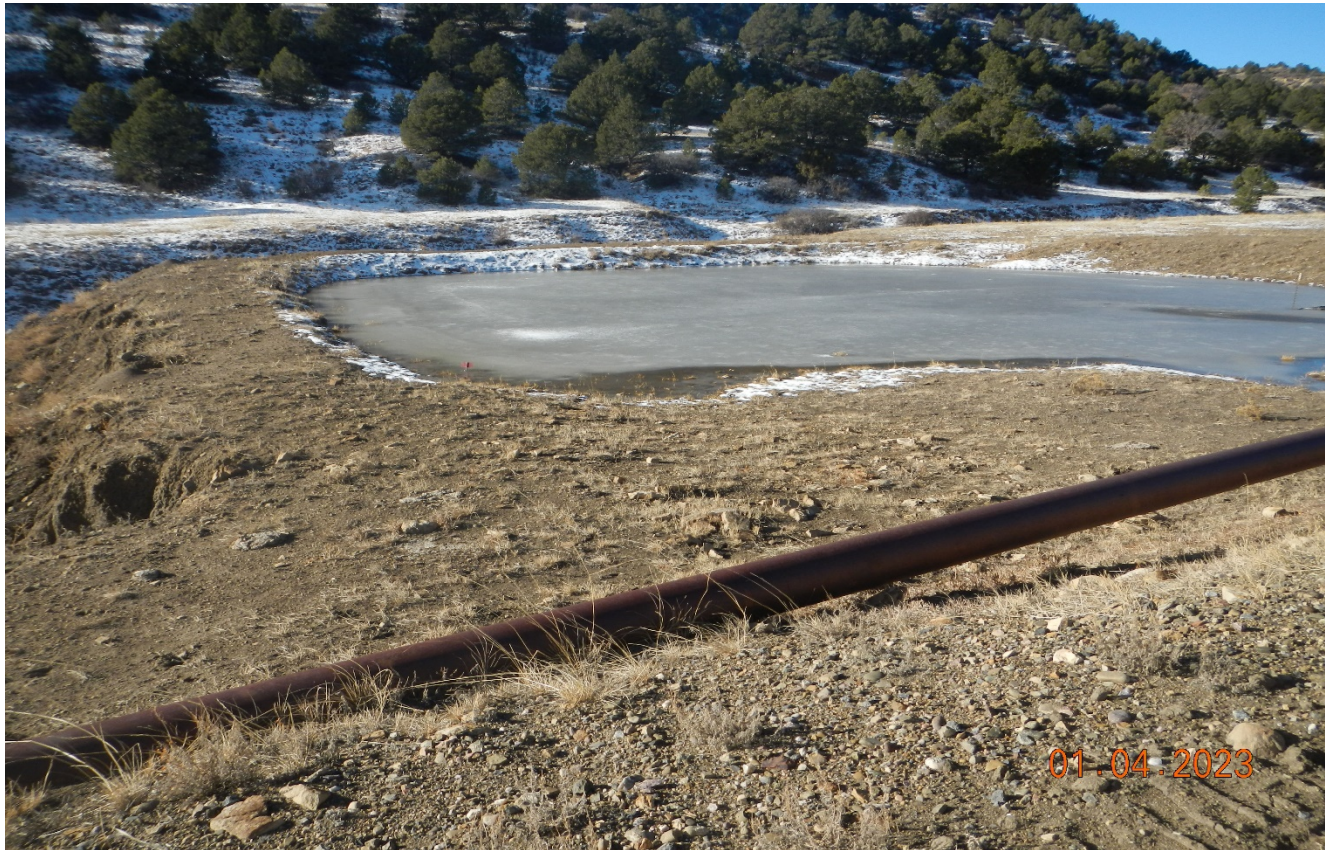
Photo 2. The water level at the pit was above 2ft. freeboard.
