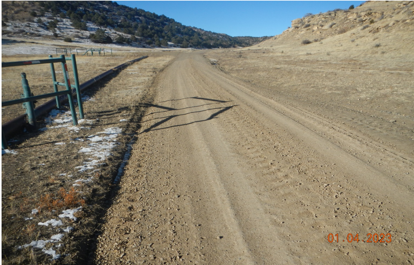
Photo 1. Facing west along the main access road. There has been additional road base applied to areas and the road was recently graded.
