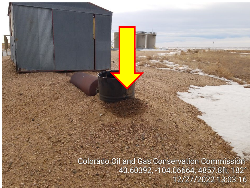
Photo 5 – Stained Soil at Exhaust
