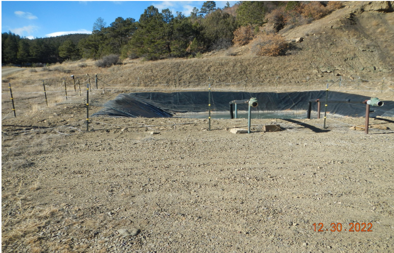
Photo 2. The electric fence is in disrepair around the pit. A more robust fencing should be considered.
