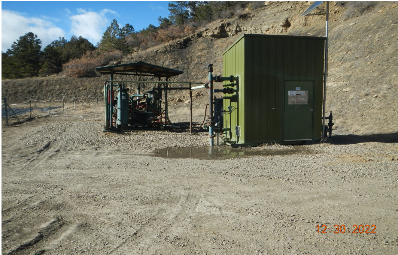
Photo 2. There is water around at the meter shed which appears to be leaking..
