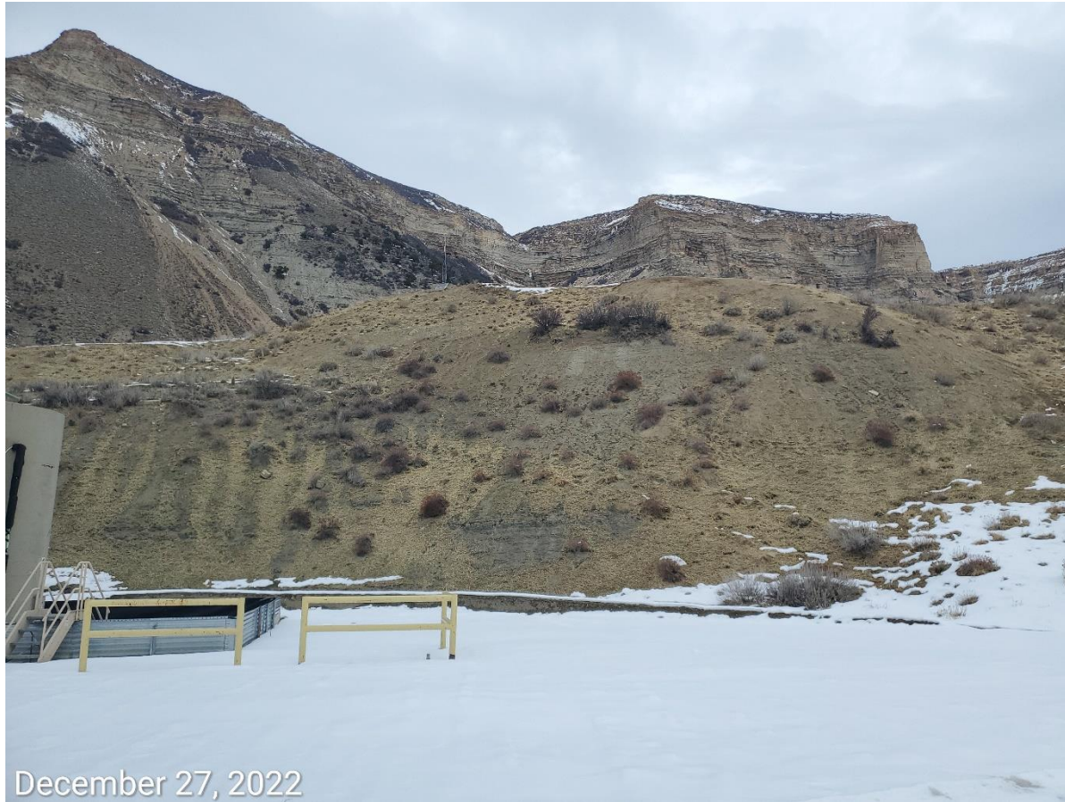
Photo 3: Photo taken from the Location, facing north. Photo shows cut-slopes of the Location. Resolution documents submitted by Operator indicate erosion was repaired, followed by an application of straw mulch and hydromulch. Photo shows large areas of the cut slope where BMPs are in disrepair, and erosion degradation is recurring: BMPs implemented have not been maintained, and do not appear to be adequate for the site's conditions
