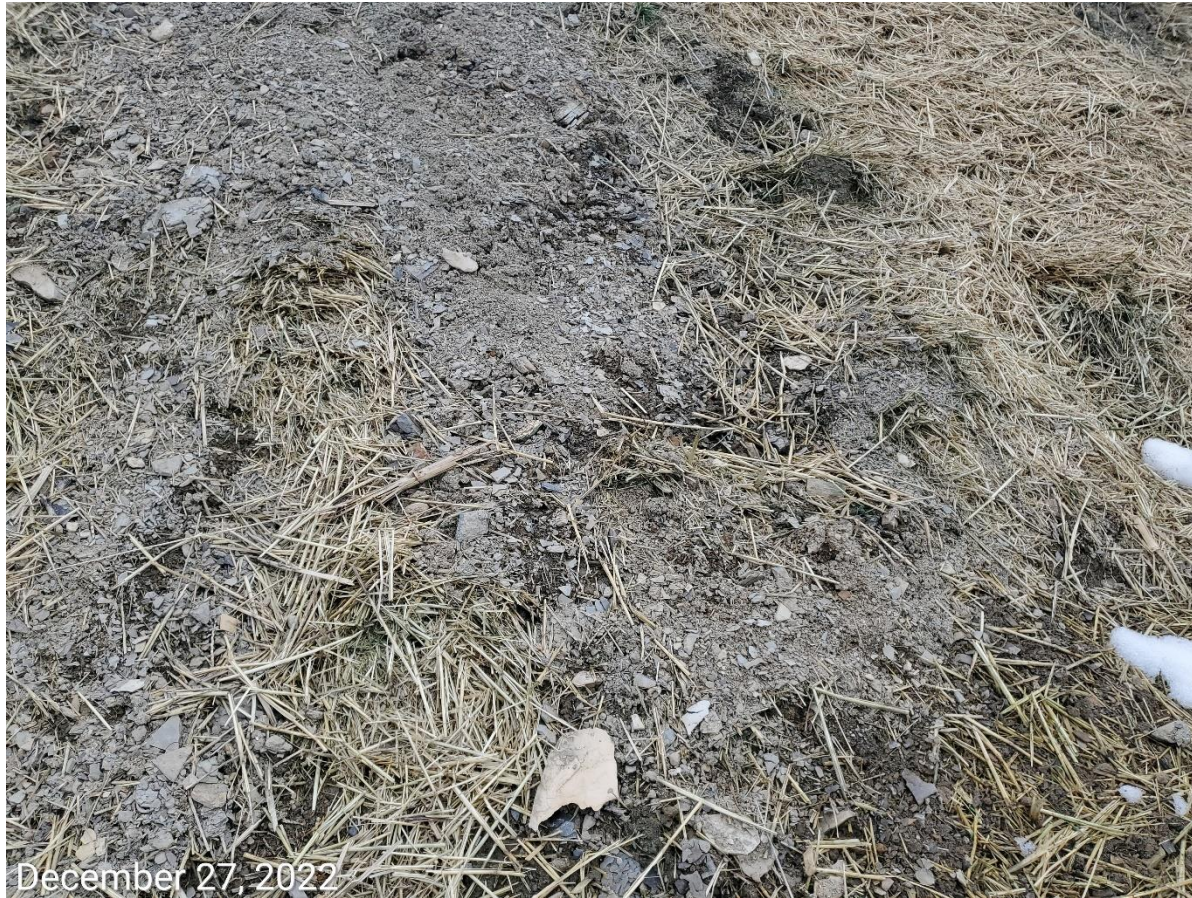
Photo 5: Photo taken from the cut slopes of the Location. Photo example showing erosion degradation at the cut slopes; specifically, photo shows sediment covering the mulch; BMPs implemented have not been maintained, and do not appear to be adequate for the site's conditions
