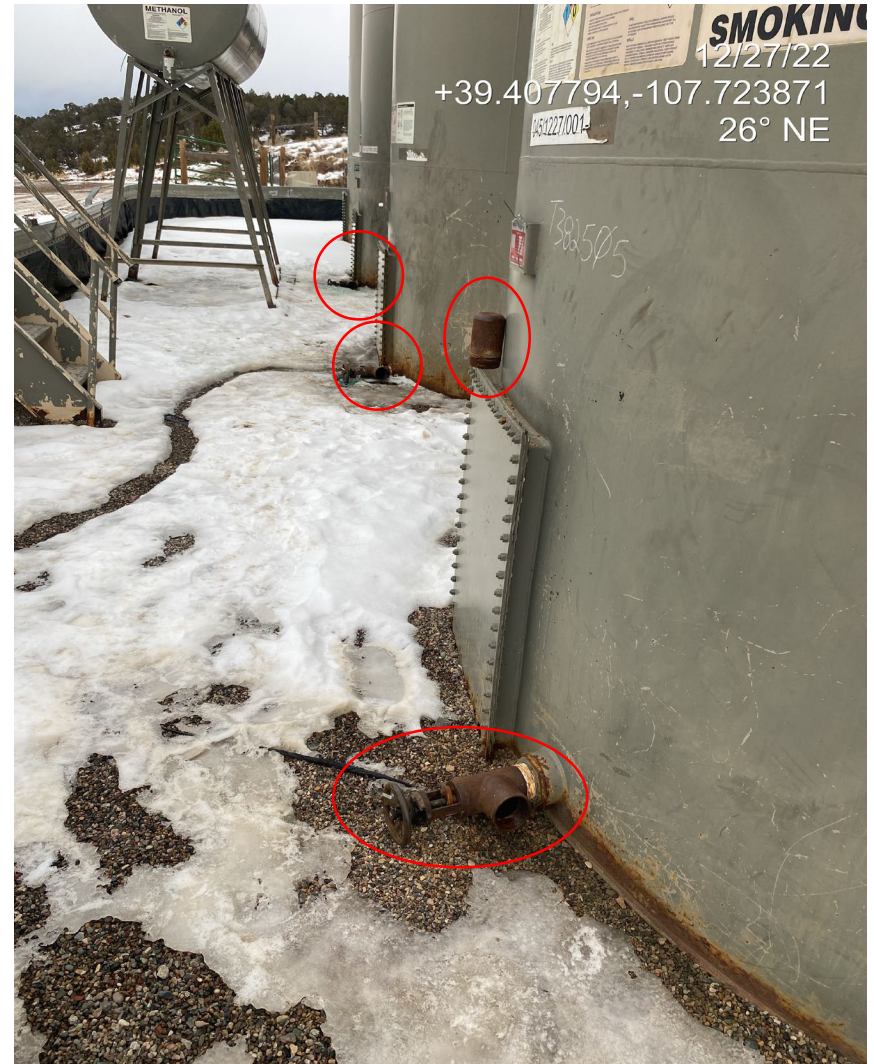
Photo 1. Photos show tank battery sign absent (left) and bull plugs not installed on tank drain lines (right).
