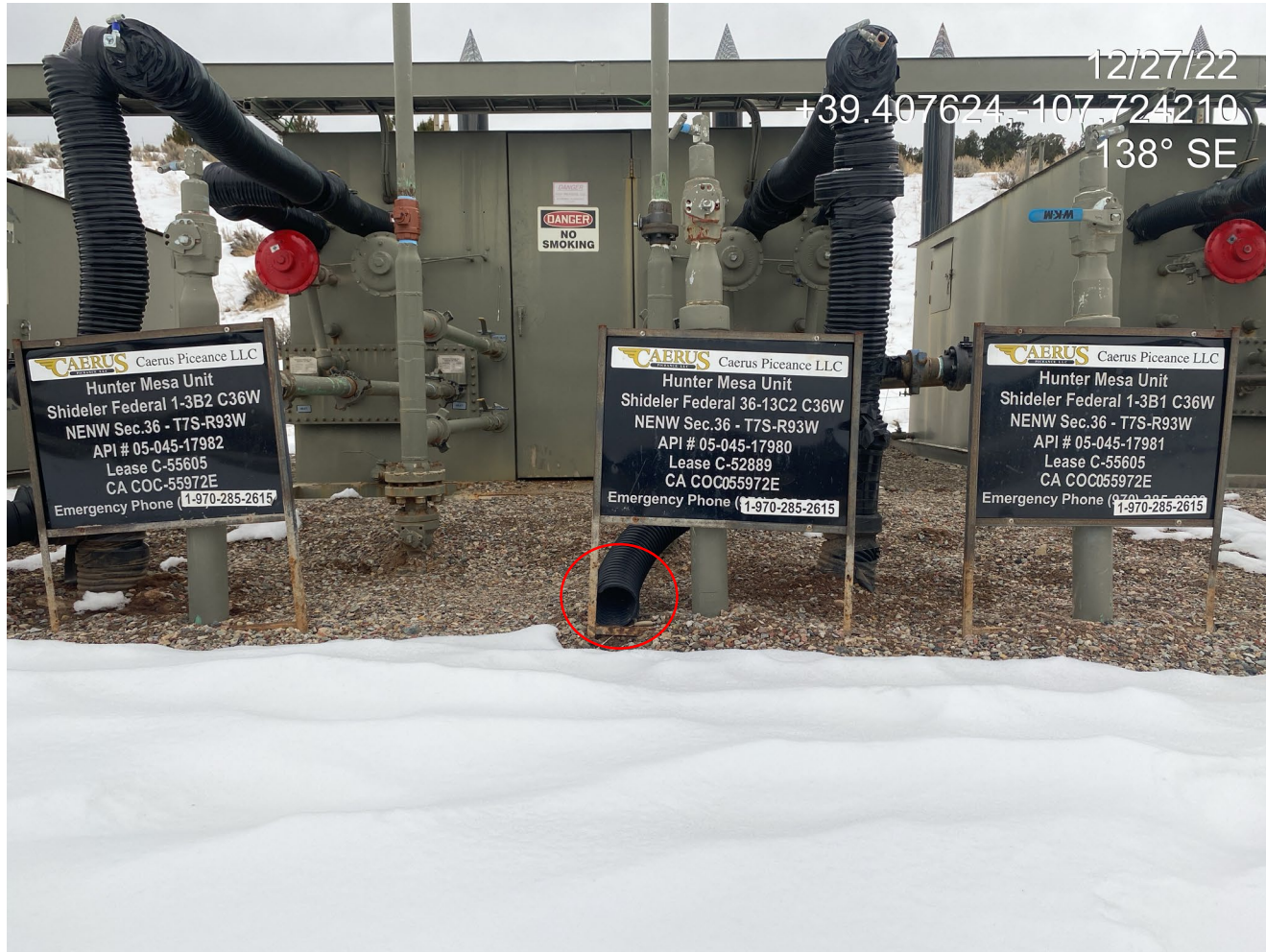
Photo 2. Photo shows open ended piping on separator line.
