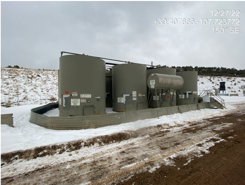
Photo 1. Photos show tank battery sign absent (left) and bull plugs not installed on tank drain lines (right).
