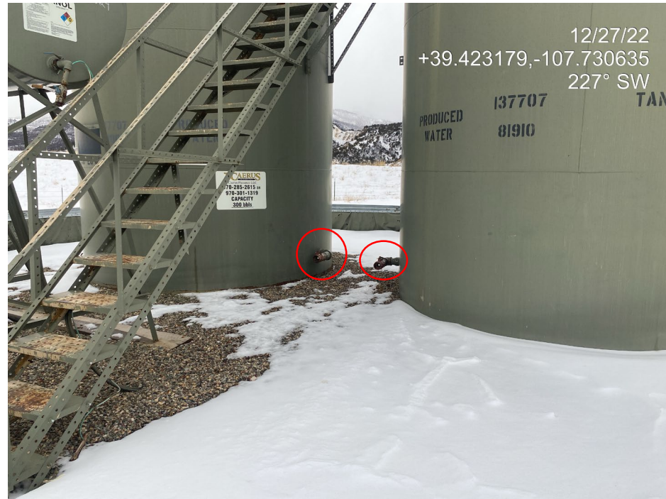
Photo 2. Photos show tank battery sign absent (left) and bull plugs not installed on tank drain lines (right).
