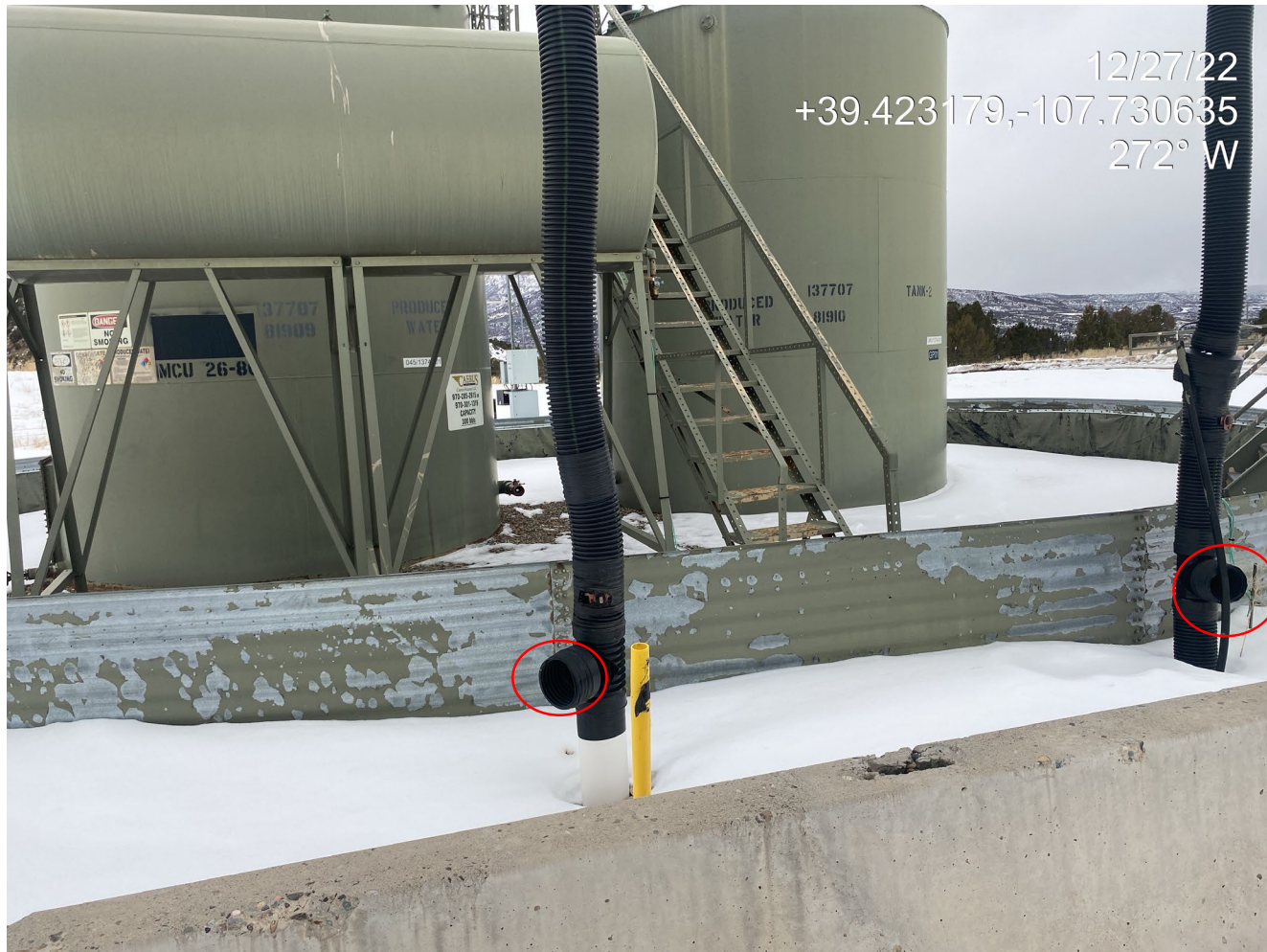
Photo 3. Photo shows open ended piping at tank battery.
