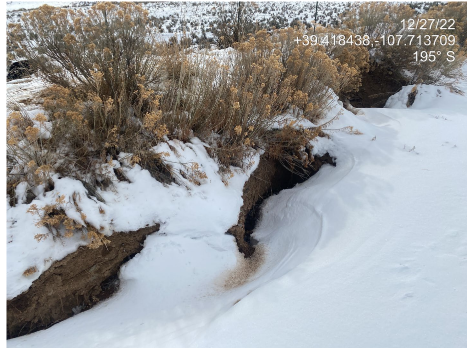
Photo 2. Photos show downward erosion/undermining of the berm at the south of the location.
