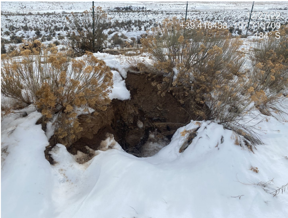
Photo 2. Photos show downward erosion/undermining of the berm at the south of the location.
