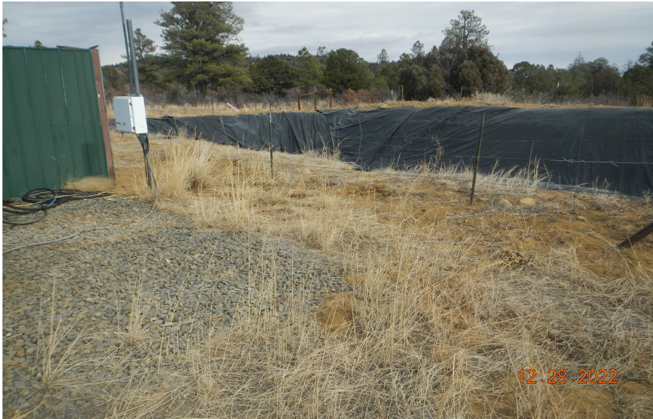
Photo 2. The stained soils have been cleaned up and fence was repaired.
