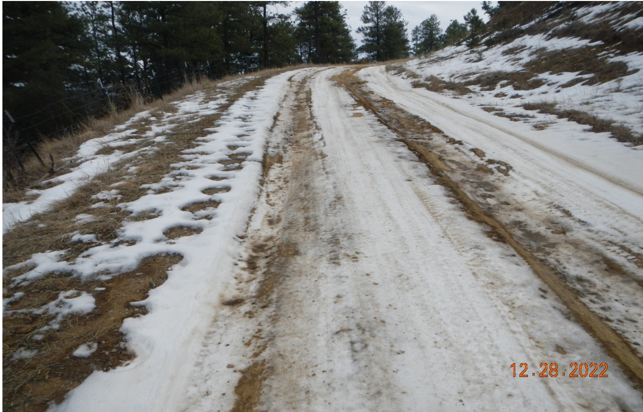
Photo 3. Further up the road there is vehicle rutting of the road. Soils are frozen so repairs will likely need to be made at a later in the season.
