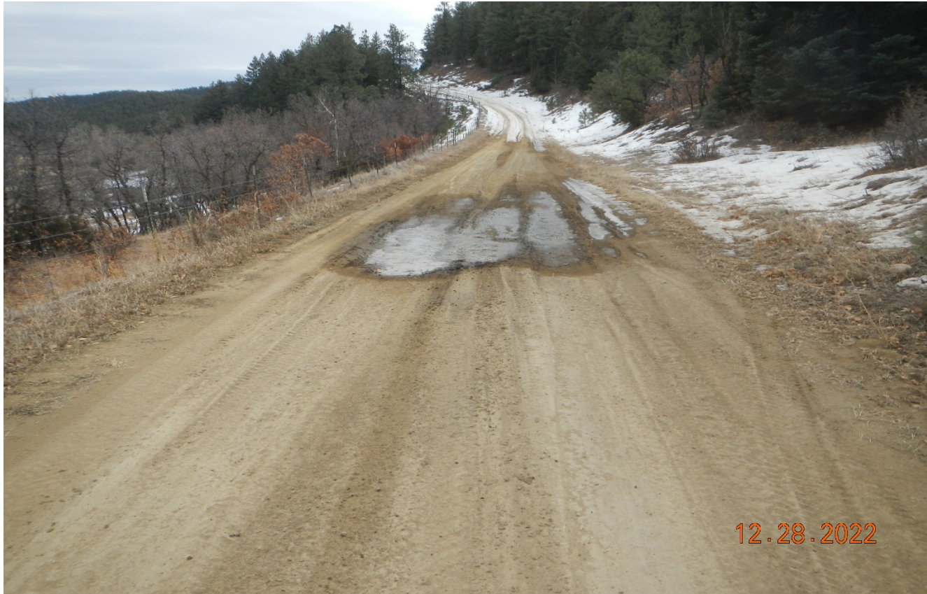
Photo 2. Facing southeast along the road. Stormwater is accumulating on the road and vehicles are driving around this area causing widening of the road. Approx. Lat/Long:37.29215,-104.84876.
