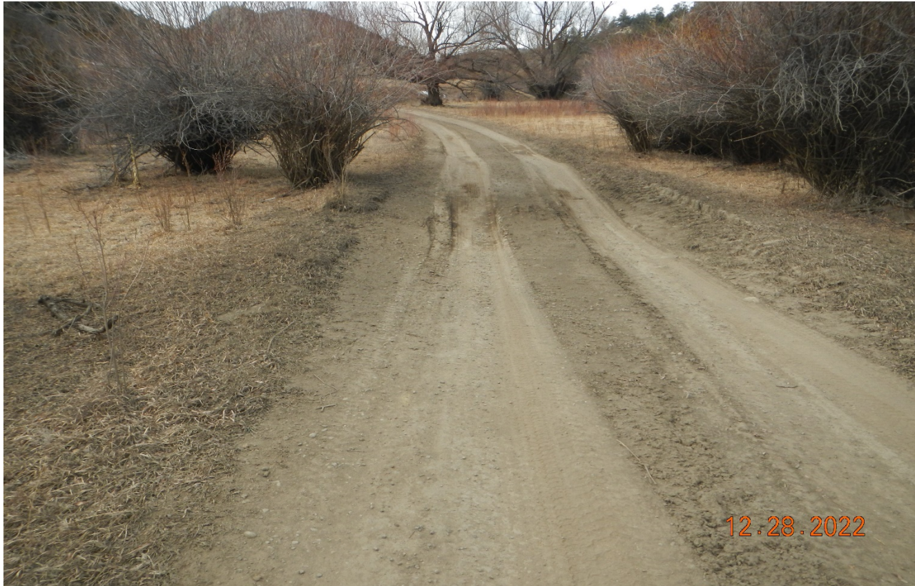
Photo 1. Facing west along the main road in Jaroso Canyon. This low area of the road accumulates the intermittent stream water and needs to be built up and stabilized. Approx. Lat/Long:37.29289,-104.84867.
