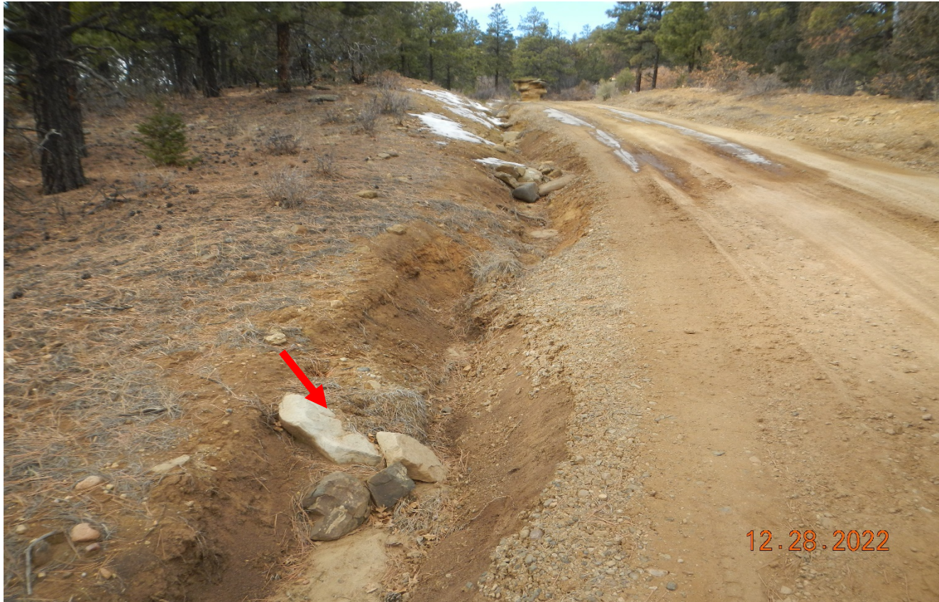
Photo 4. Facing northwest along the main road. The rock check dams are in need of maintenance. Lat/Long:37.28628,-104.85538.
