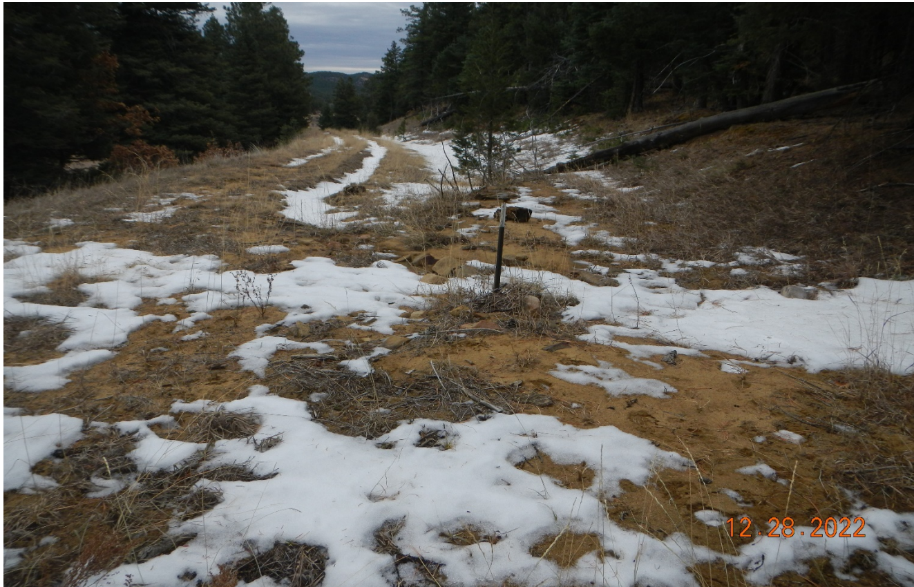
Photo 1. Facing east along the pre-existing access road. This culvert has filled in with sediment causing stormwater to flow down the road causing erosion.
