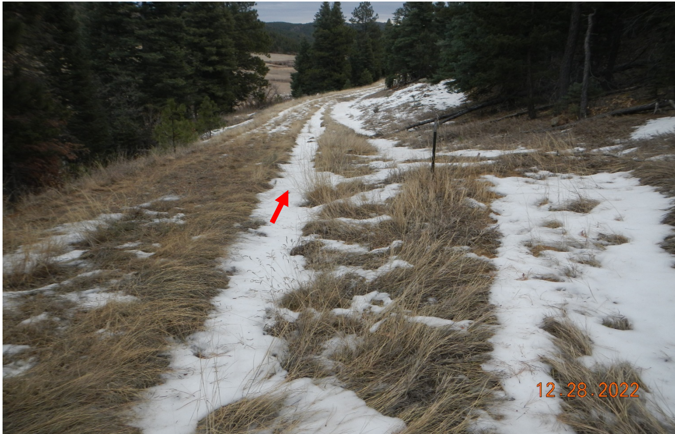
Photo 2. Another culvert further down the road has filled in with sediment. There is erosion along the road shown at red arrow.
