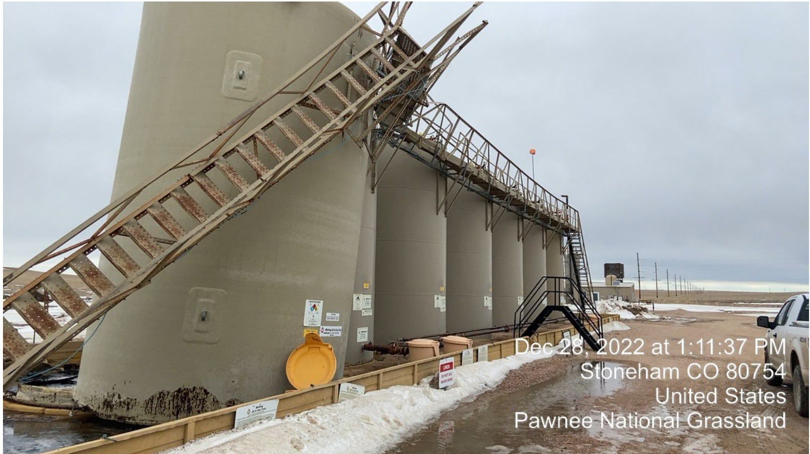
Damaged Produced Water Tank
