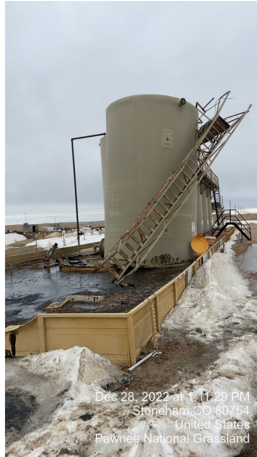
Damaged Produced Water Tank
