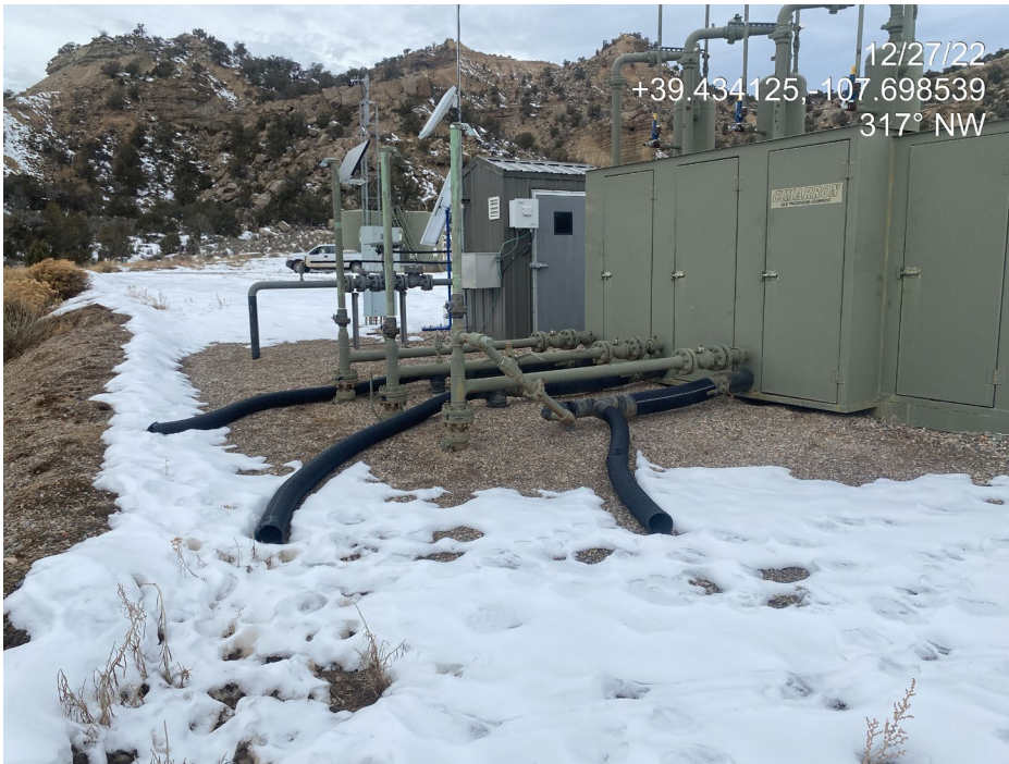
Photo 3. Photos show open ended piping at separators (left) and tank battery (right).
