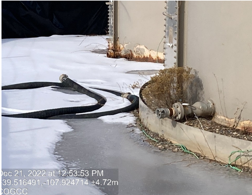
Lines on tanks missing caps/plugs
