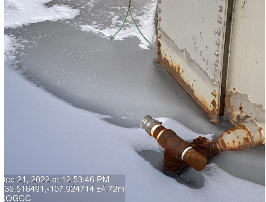
Lines on tanks missing caps/plugs
