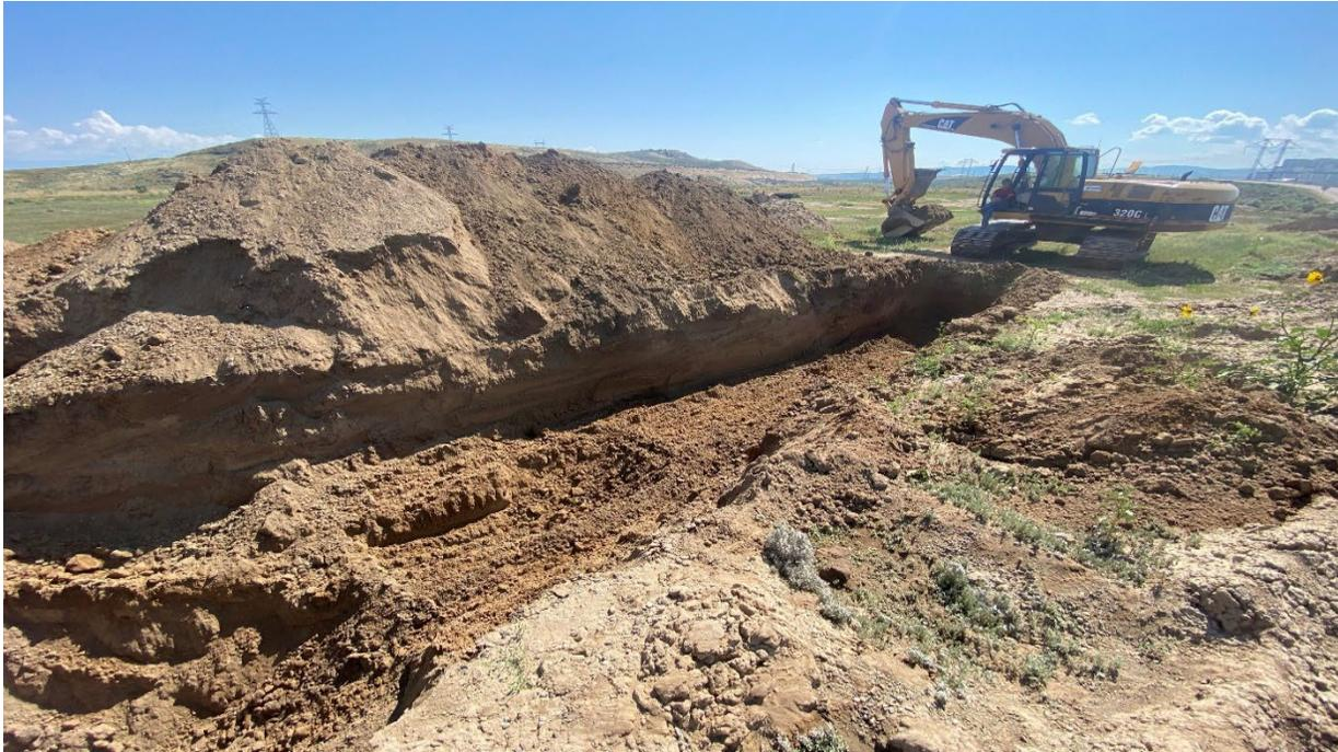
Excavation continued southeast for ~30 feet, from ~9 feet BGS gradually decreasing in depth to ~6' BGS until the south side wall and entire excavation bottom were screened using a PID and all samples were < 100 ppm VOC. Eight (8) confirmation samples were collected from the excavation bottom and side walls.
