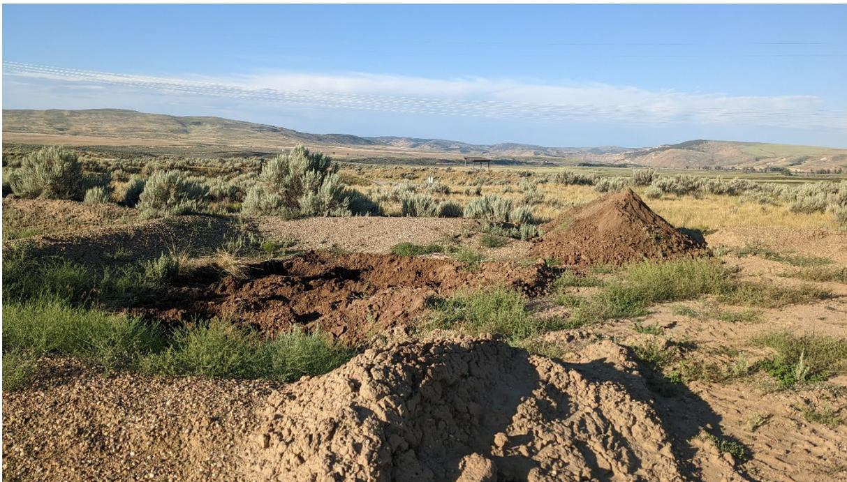
TCO then excavated in the former tank battery working toward the southeast secondary containment. until the excavation was ~9 feet BGS. The excavated bottom and side walls were screened using a PID and all samples were > 100 ppm VOC. Further excavation was postponed until a track hoe could be transported on site. The excavation pit was covered with a tarp to avoid precipitation leaching contamination deeper in soil.
