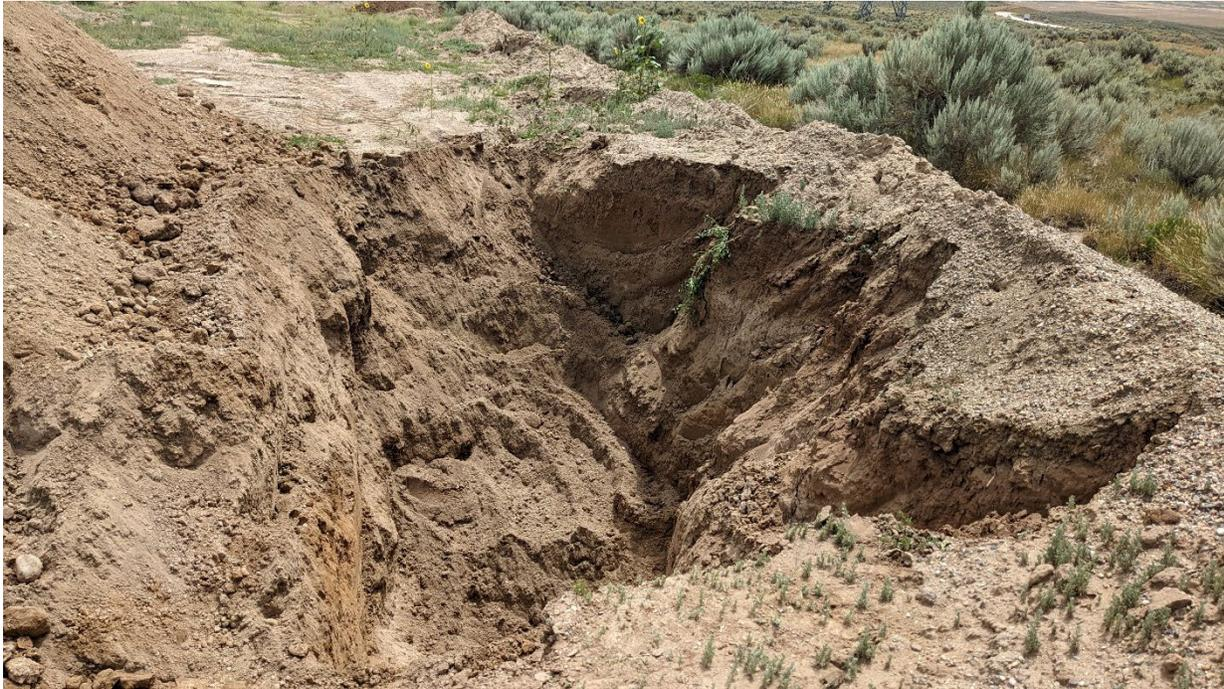
TCO excavated around the former wellhead. Three soil stains were observed on the surface near the wellhead (R\_WH) and soil piles. Each stain location was excavated and the area around the wellhead was excavated too. The excavation bottom and side walls were screened with PID readings < 100 ppm. Four (4) confirmation samples were collected from the excavation bottom and side walls.
