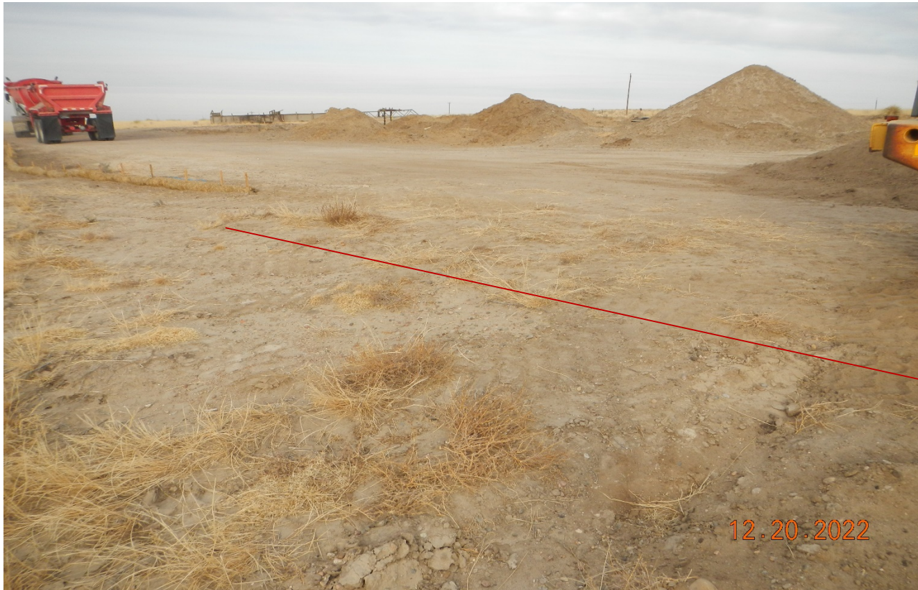
Photo 5. Facing north at the southwest side of the tank battery location. Additional BMP's should be installed on the down gradient side shown at red line down gradient of soil stock pile.
