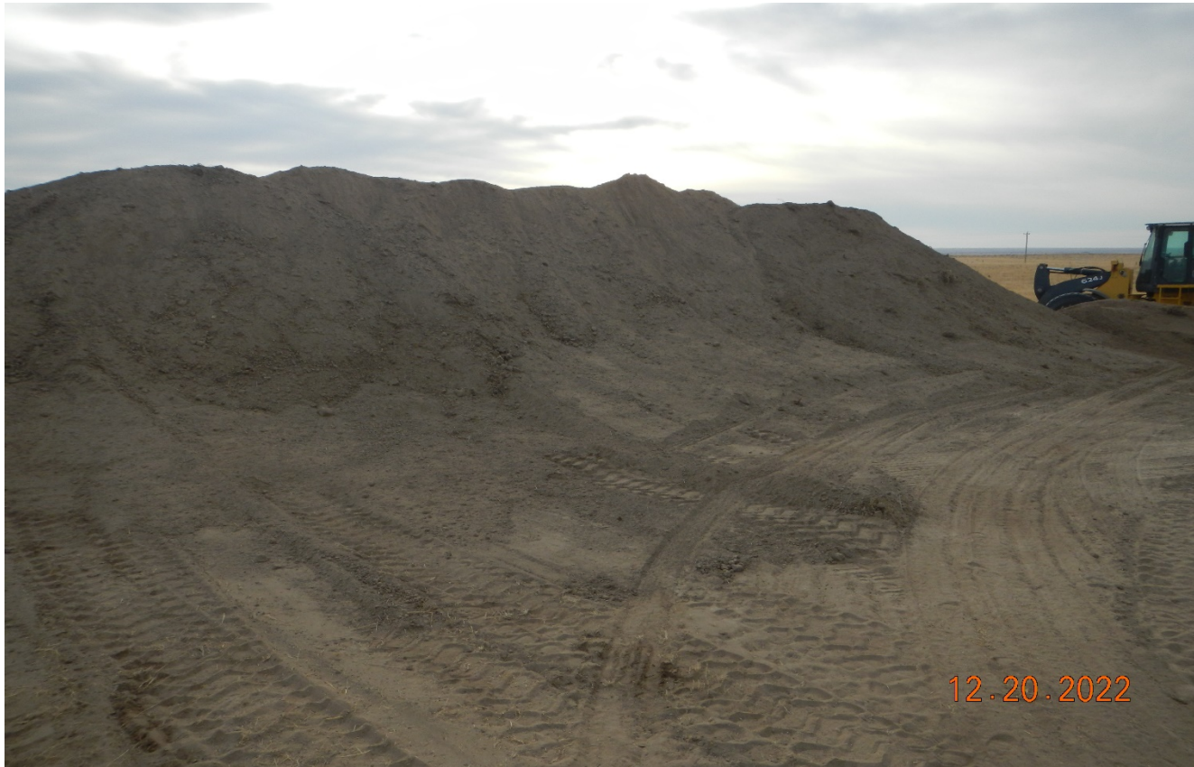
Photo 4. Facing toward the south side of the location. Soil is being hauled in and stored on the location. Temporary erosion controls will be need to prevent erosion of the loose soils.
