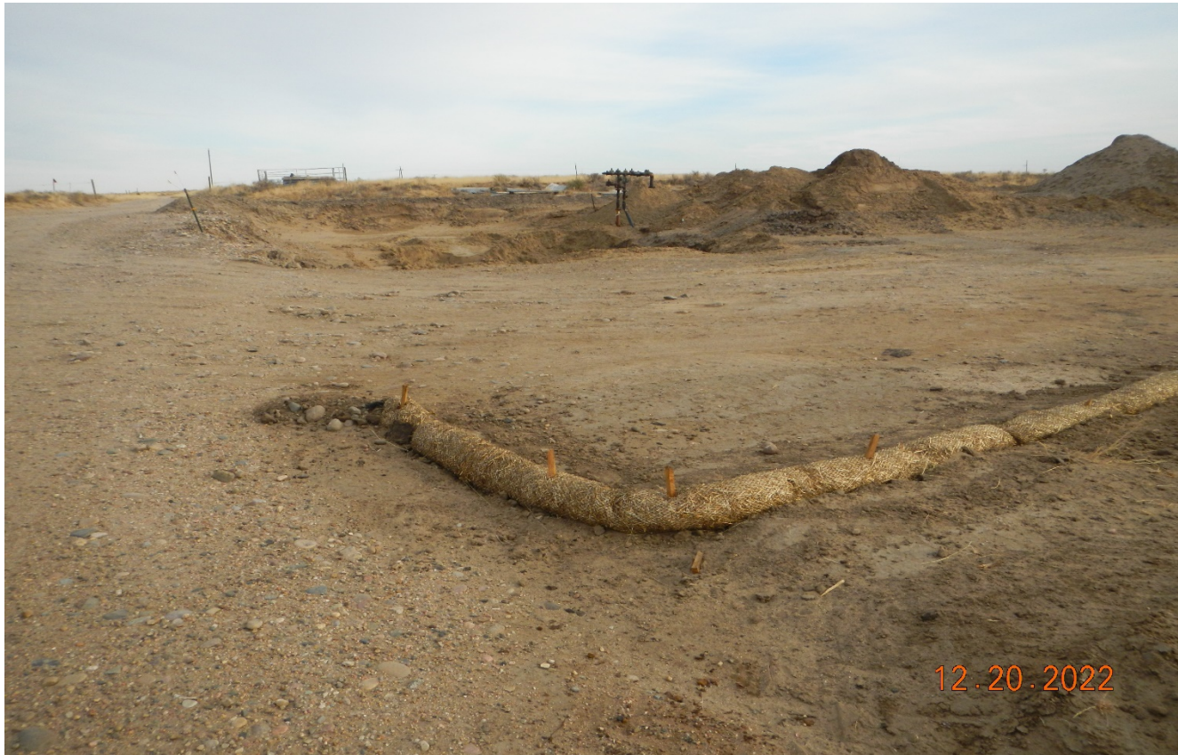
Photo 3. Facing southeast toward the tank battery location. Straw wattles have been installed along the west side of the location.
