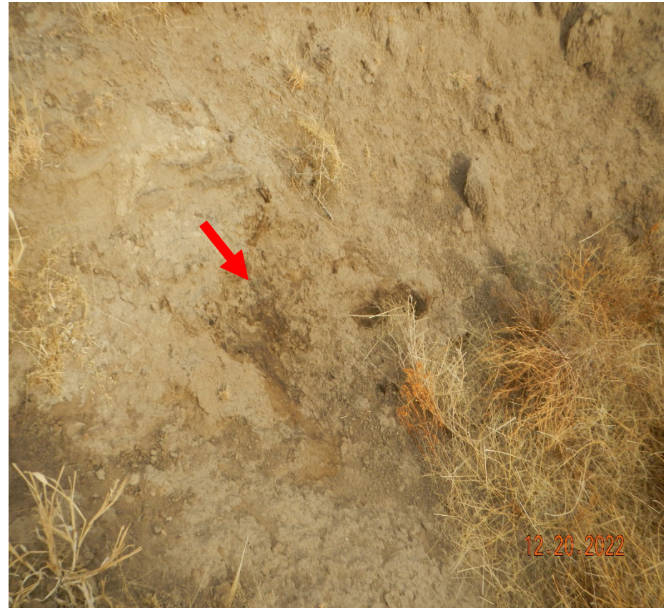
Photo 7. Located at the western side of the spill area. There is an excavated hole at this area approximately 12'x12'6'. There are still areas of oil stained soils at the surface (Bottom left) and 2ft. Down into the excavation area (right photo). Further excavation is needed.
