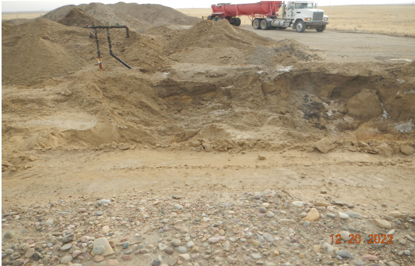
Photo 1. Facing south toward the tank battery facility. The tank was removed and soils have been excavated in this area. Remediation project: 20712
