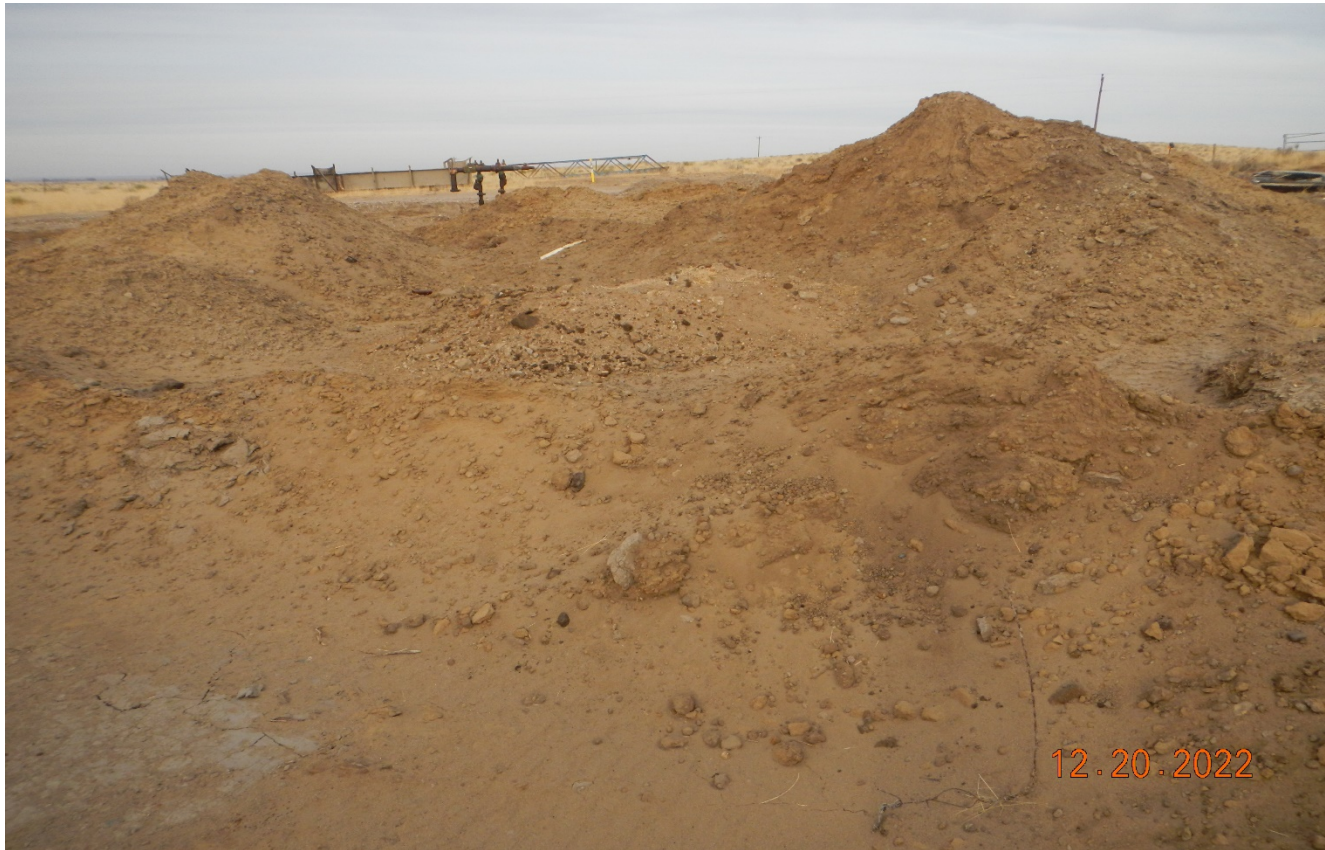
Photo 2. The berms around the soil piles have been constructed larger but were not compacted. Also, no liner was observed under the contaminated soils. Contaminated soils should be removed and properly disposed ASAP.
