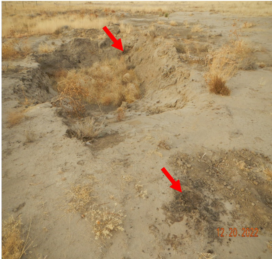
Photo 7. Located at the western side of the spill area. There is an excavated hole at this area approximately 12'x12'6'. There are still areas of oil stained soils at the surface (Bottom left) and 2ft. Down into the excavation area (right photo). Further excavation is needed.
