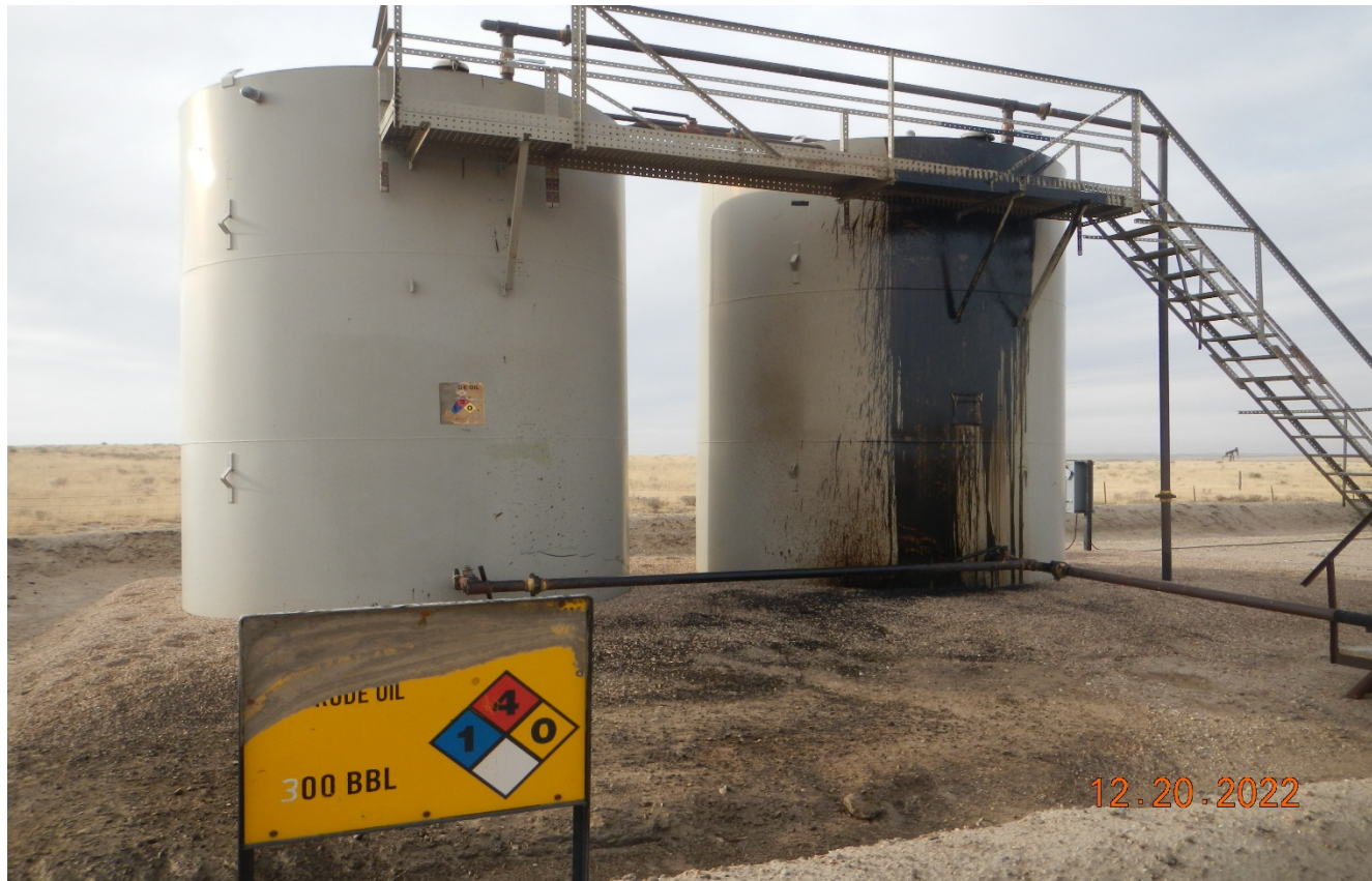
Photo 1. Facing toward the tank battery. It appears a recent spill occurred at the tank contained inside the bermed area. Stained soils need to be cleaned up and removed.
