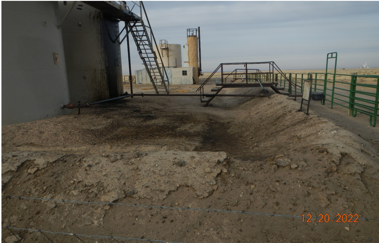
Photo 2. It appears a recent spill occurred at the tank contained inside the bermed area. Stained soils need to be cleaned up and removed.
