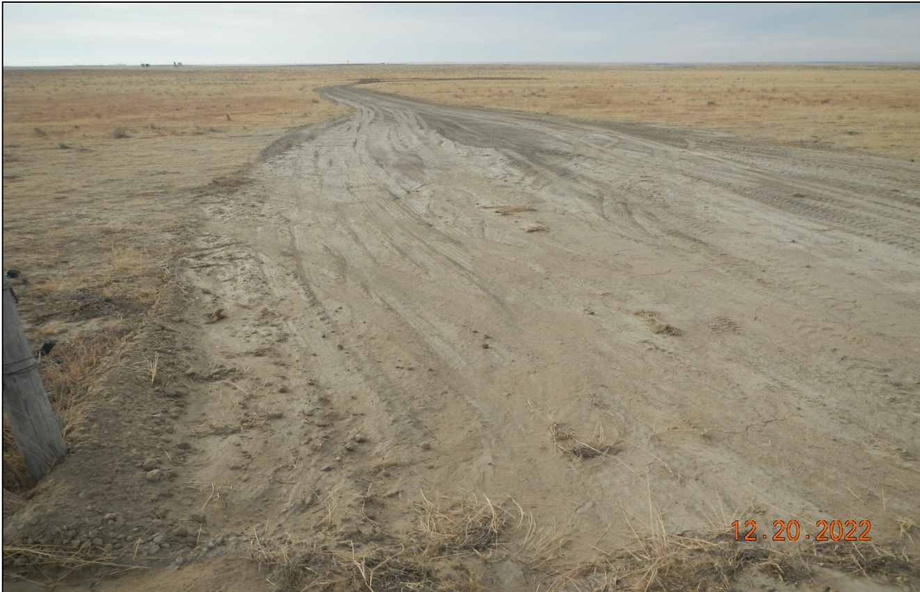
Photo 1. Facing west at the beginning of the access road. The cattleguard has been removed and the road regraded. It does not appear reclamation including seeding has been completed.
