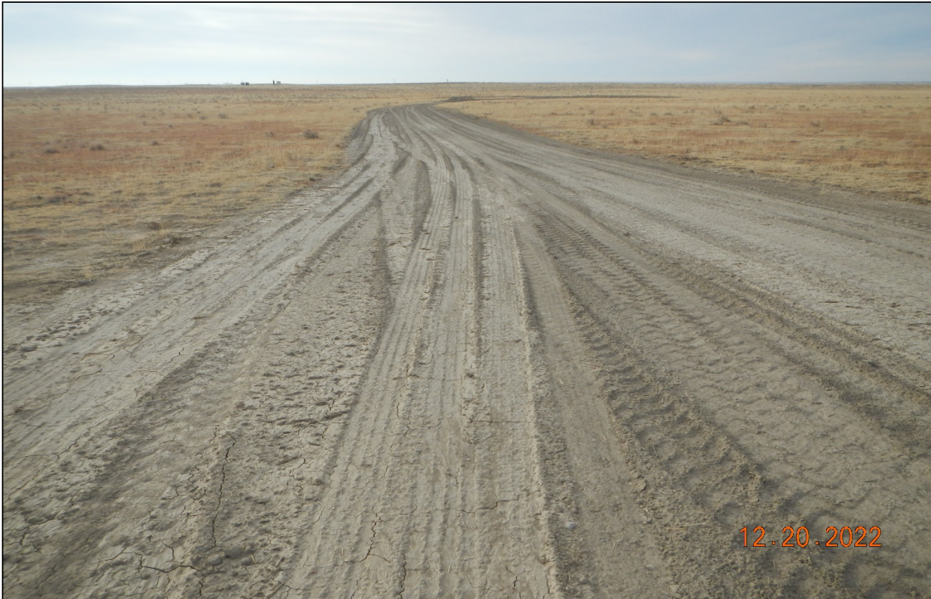
Photo 2. Facing west toward the access road. This area needs to be leveled out and reclaimed. It does not appears reclamation including seeding has been completed.
