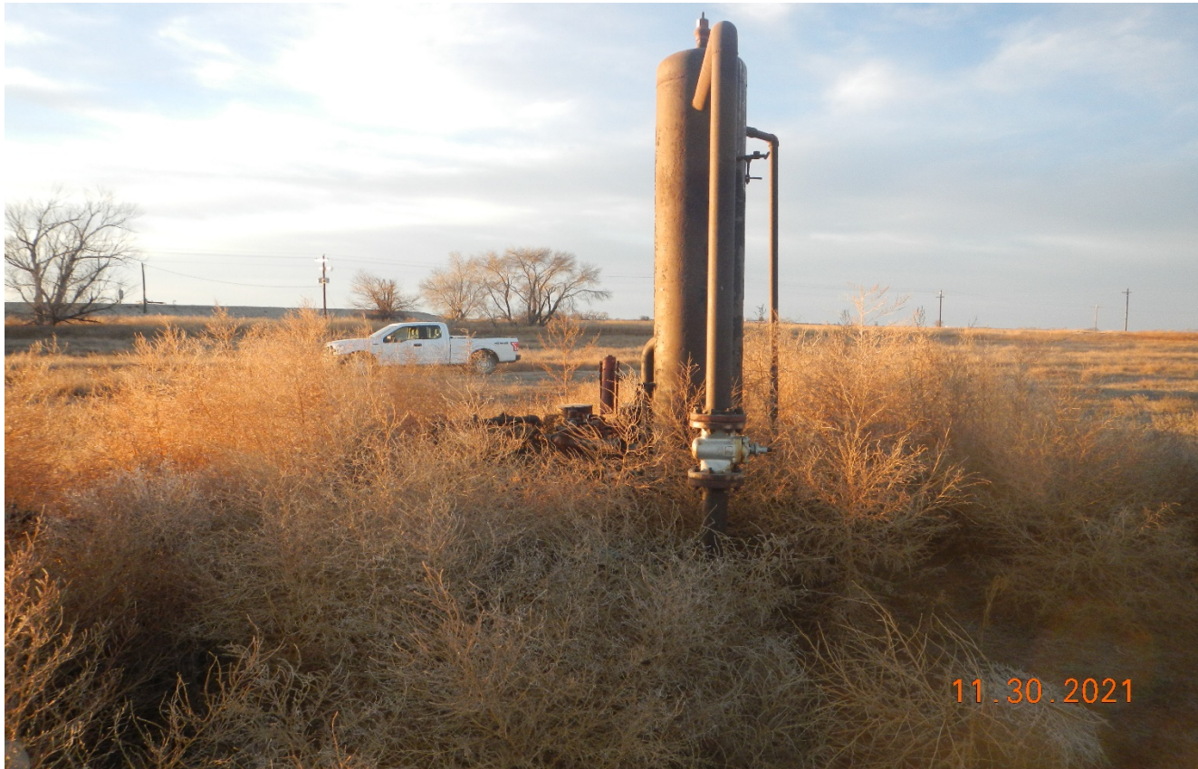
Photo 3. Facing west. There is abandoned gas separator that remains at the location. There is also undesirable weeds growing around the abandoned equipment. Previous corrective action was not completed. Photo taken 11/30/21.
