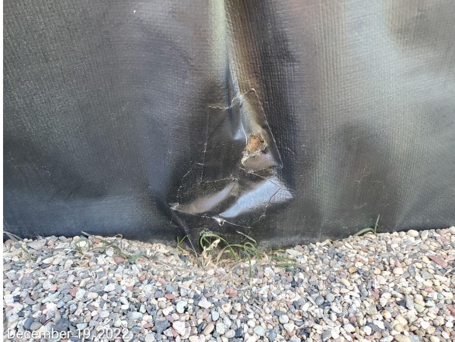
Photo 5: Photos examples showing various holes observed throughout the entire liner at the tank battery.
