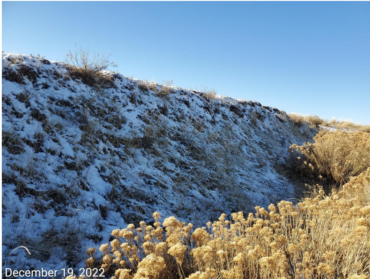
Photo 3: Photo shows cut slopes on the south end of the Location- slopes appear to be vegetated and stabilized.
