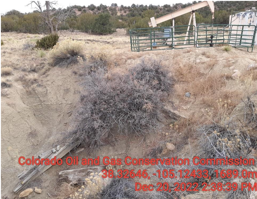
Photo 3 Storm water erosion near well head
