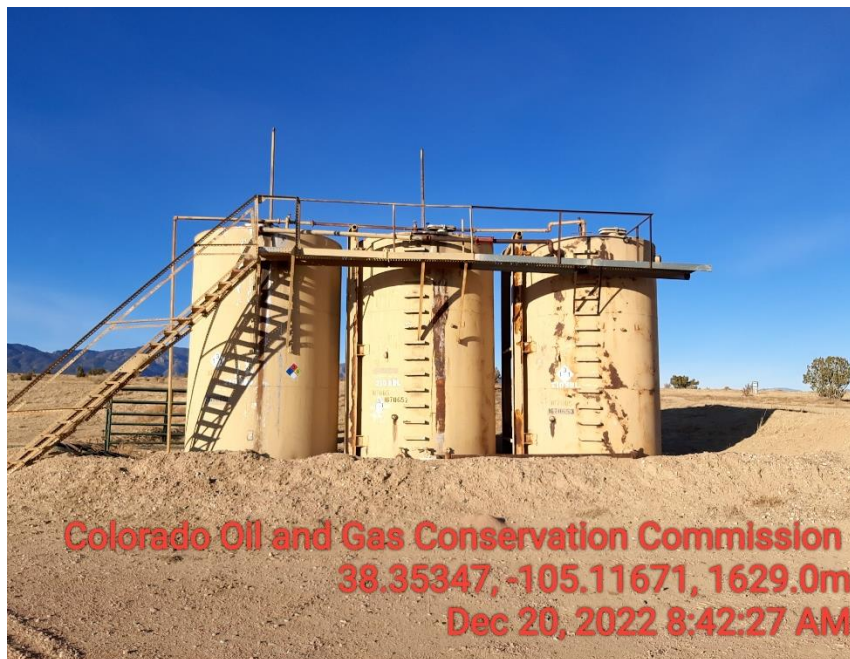
Photo 1 TNK BTRY No battery sign, No NFPA placards on two tanks
