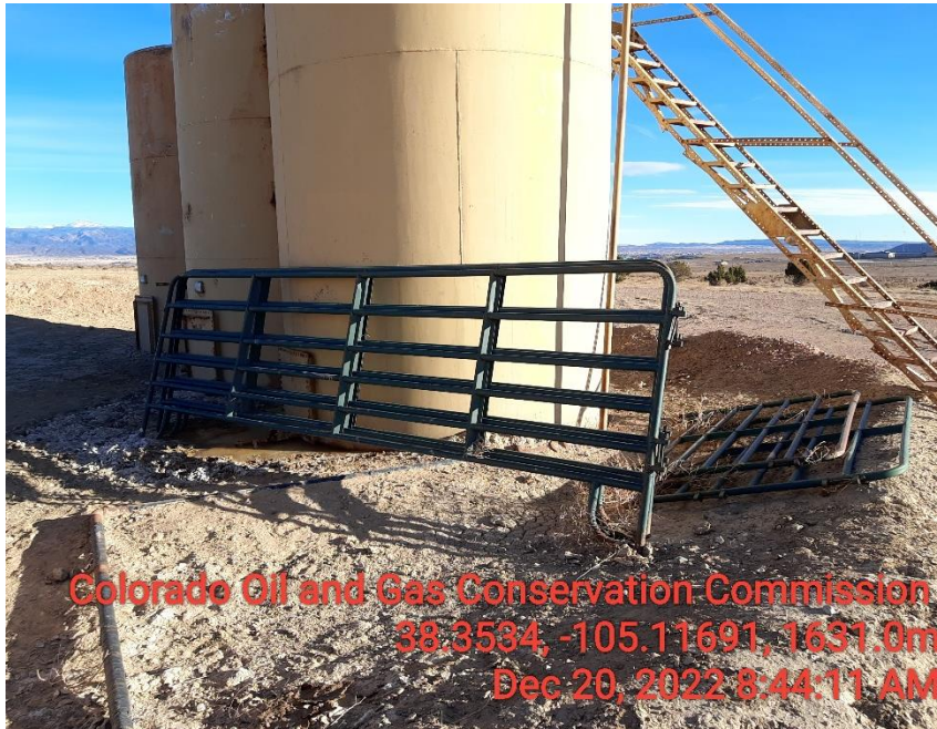
Photo 3 unused equipment: cattle panels in crude oil containment area
