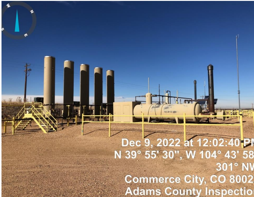
Photo#3 Separators/ECD's/Automation RTU
