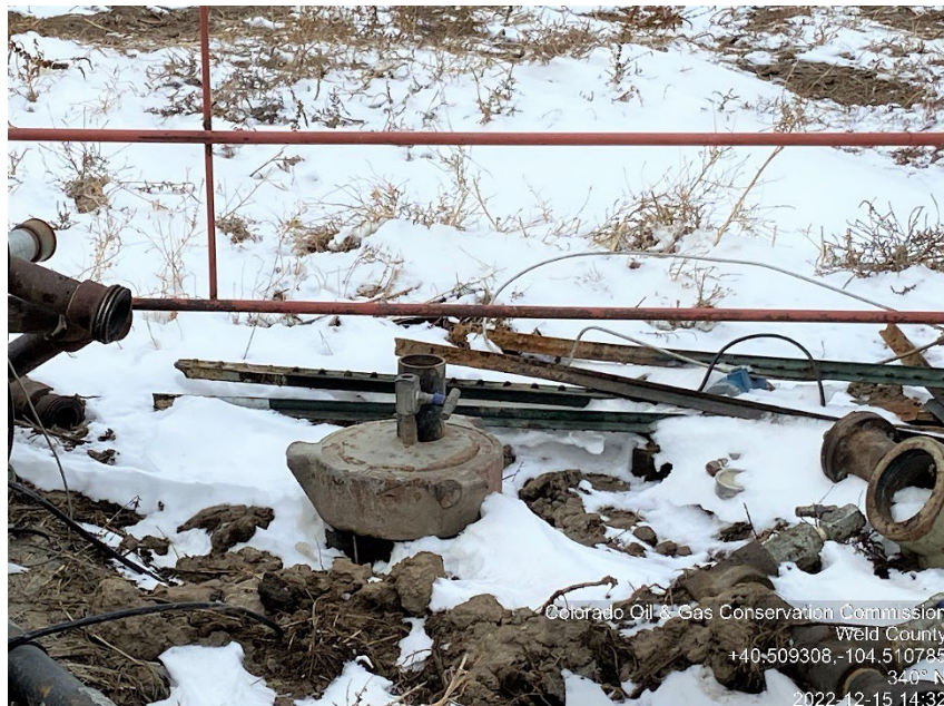
Photo #1 Pettinger 44-2 (123-22572) Wellsite Plugged & Abandoned | PA NOT cut / capped
