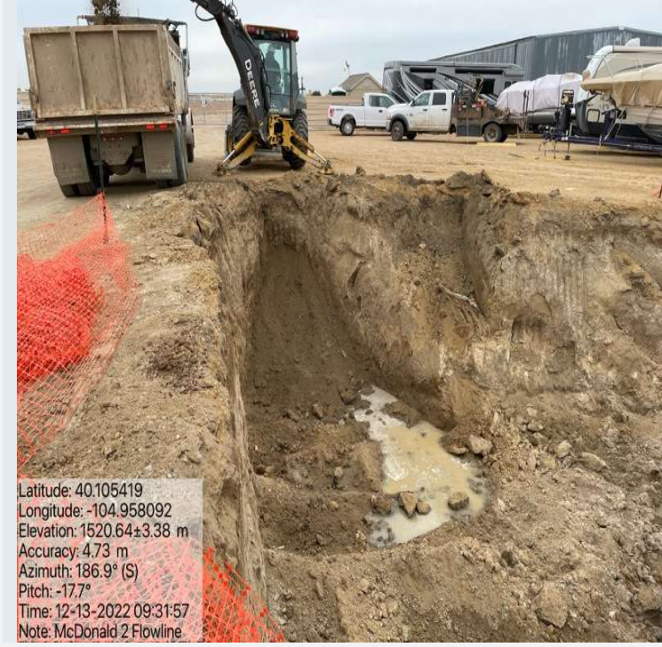
General Site - McDonald 2 Flowline
