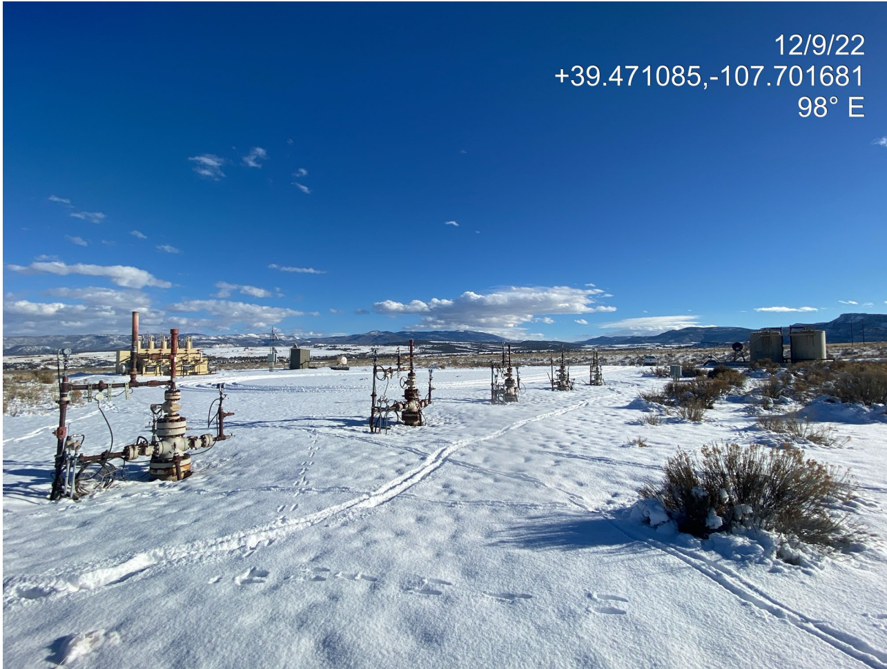
Photo 1. Photo taken from the west shows an overview of the location.
