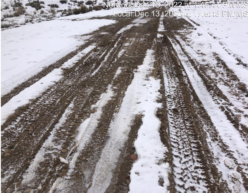
Photo #8674 Insufficient tracking BMP at entrance to location.
