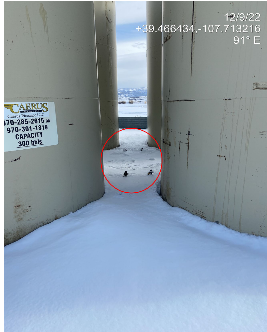
Photo 1. Photo shows four (4) LOTO risers within the tank battery. Unused riser equipment must be removed.
