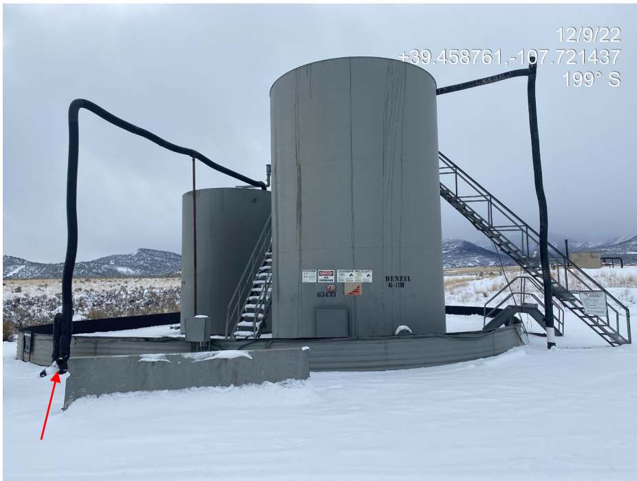
Photo 4. Photos show BMPs to prevent wildlife access to piping at tank battery are absent.
