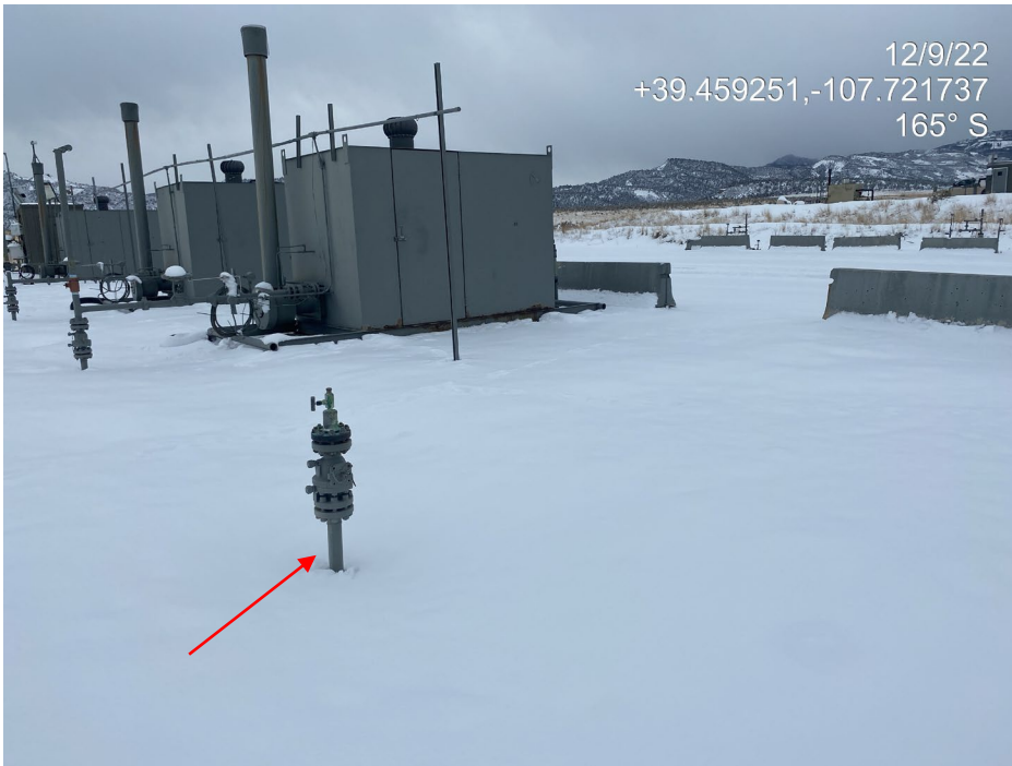
Photo 3. Photos show unused equipment (two (2) risers) at the separators at the northeast of the lower production pad.
