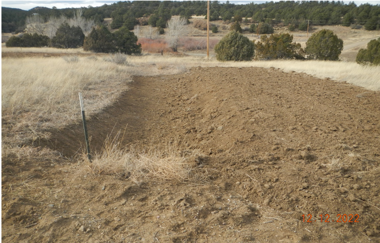
Photo 3. This culvert outlet along the road has been cleaned out and soils were seeded. Outlet protection should be installed to prevent erosion.
