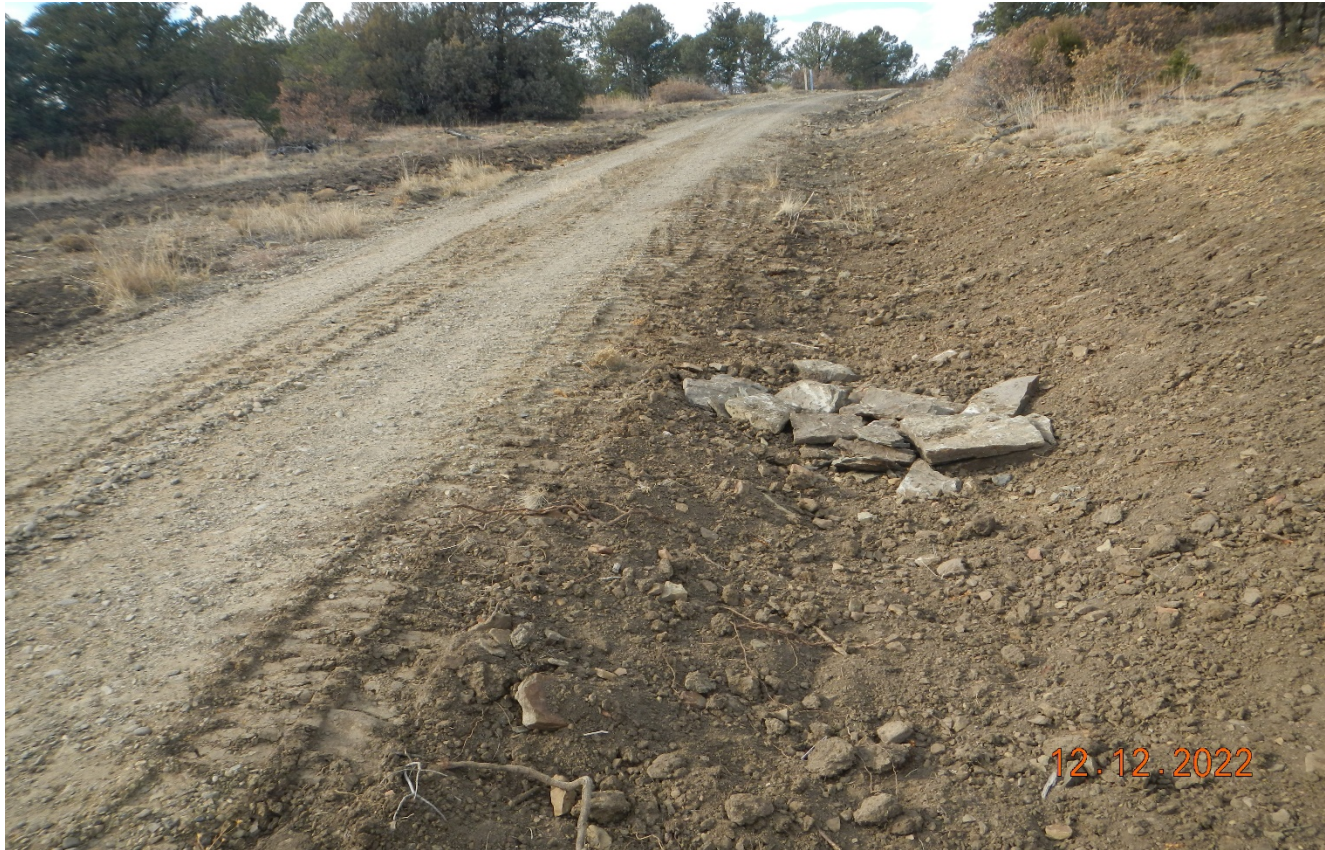
Photo 6. Facing northeast along the access road. Repairs have recently been performed along the road. The check dam is not sufficiently installed and more BMP's are needed in this area. Does not appears disturbed soils were seeded.
