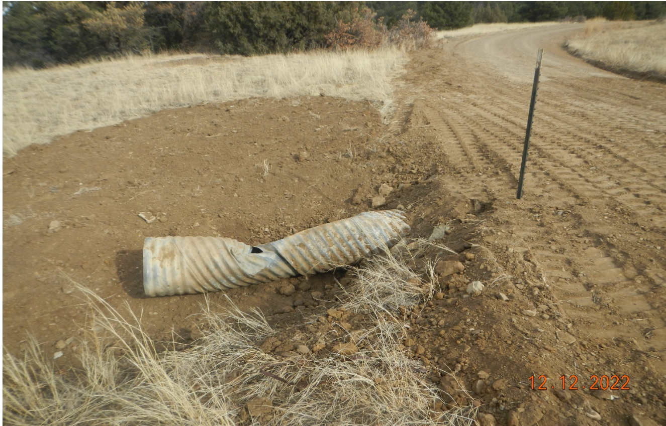
Photo 4. This culvert along the road has been cleaned out however the damage portion needs to be cut off so it doesn't plug up with sediment.
