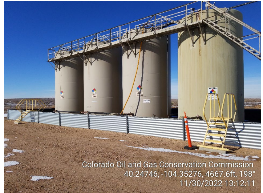
Photo 4 – Tank Battery
