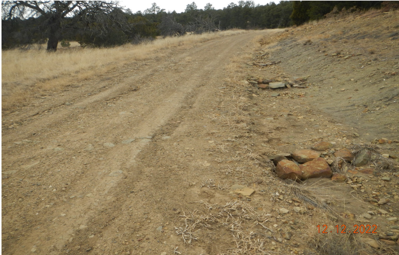
Photo 2. Facing northwest along the access road. The rock check dams have filled in with sediment and are in need of maintenance.
