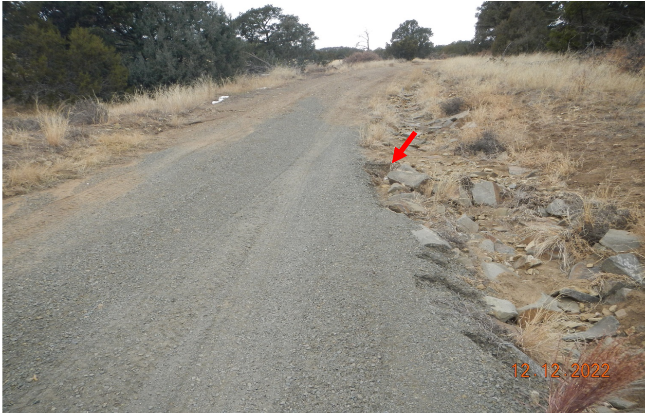
Photo 1. Facing west at the beginning of the access road. Stormwater is flowing around the rock check dam at the red arrow and is in need of maintenance.
