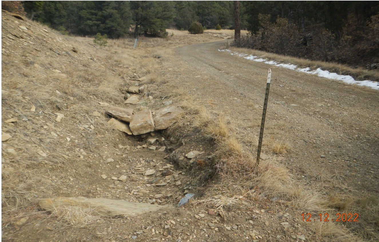
Photo 1. The culverts along the road have been maintained.
