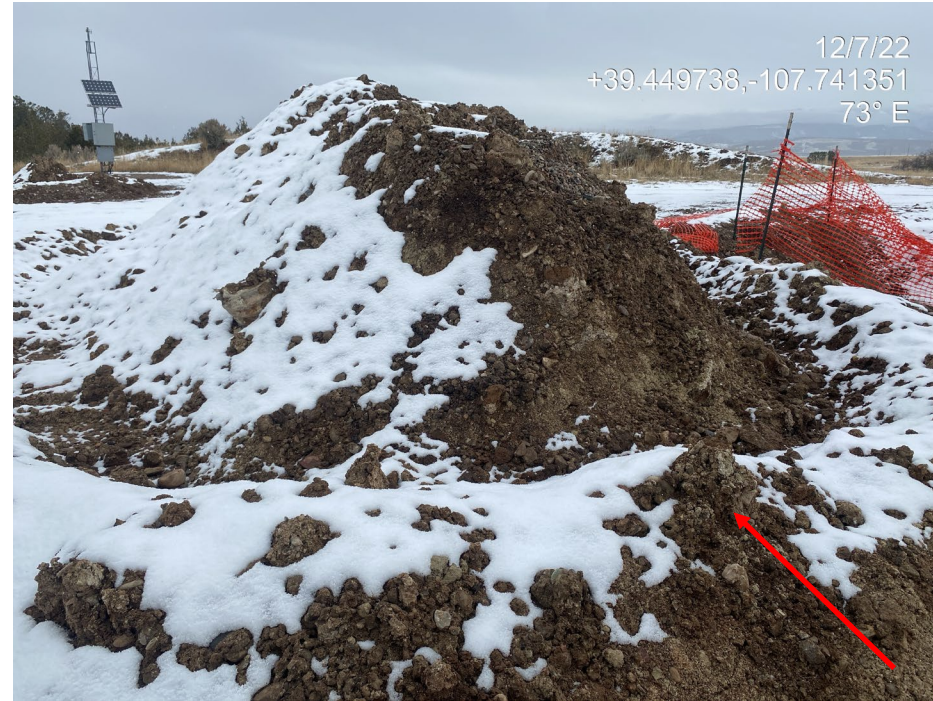
Photo 4. Photos an excavation at well API #045-10247. Excavated soil is surrounded by a berm of loose, unconsolidated soil. Orange safety fence is in disrepair/not properly installed to exclude entry into trench.
