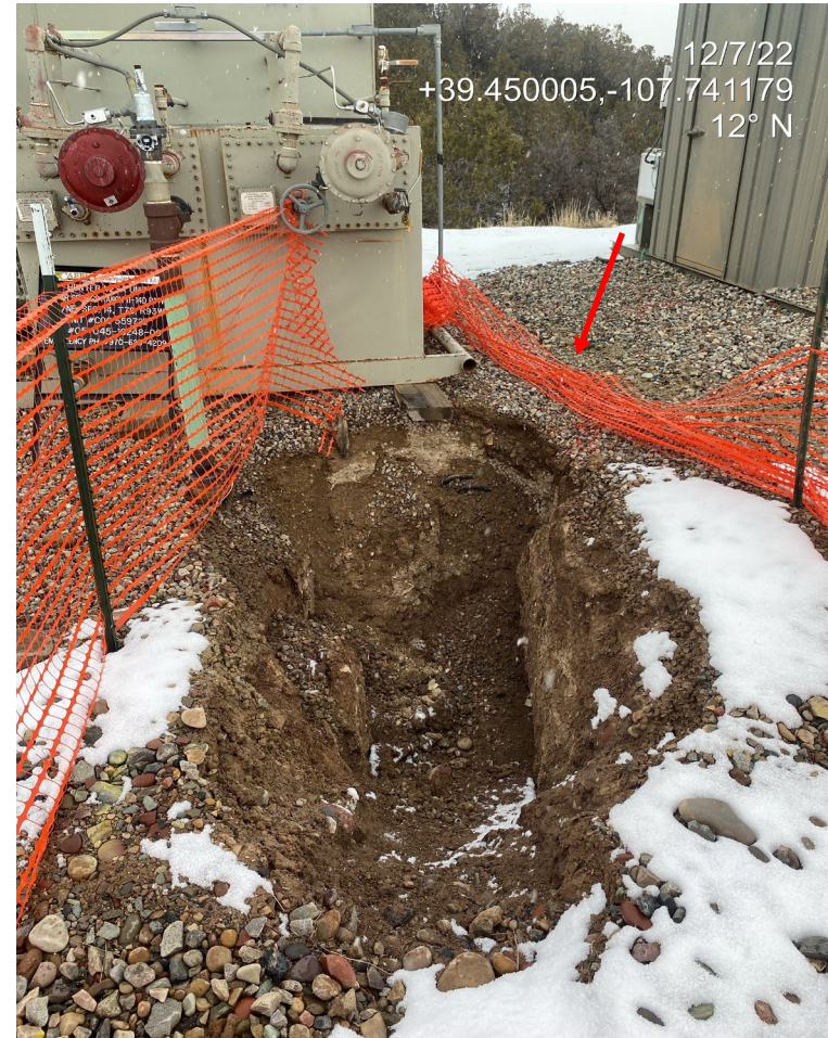
Photo 3. Photos show production areas and an excavation at separators. Excavated soil is surrounded by a berm of loose, unconsolidated soil. Orange safety fence is in disrepair/not properly installed to exclude entry into trench.
