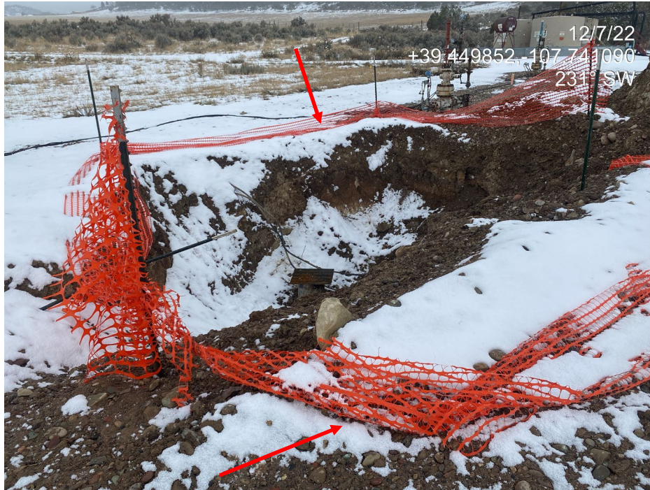
Photo 4. Photos an excavation at well API #045-10247. Excavated soil is surrounded by a berm of loose, unconsolidated soil. Orange safety fence is in disrepair/not properly installed to exclude entry into trench.
