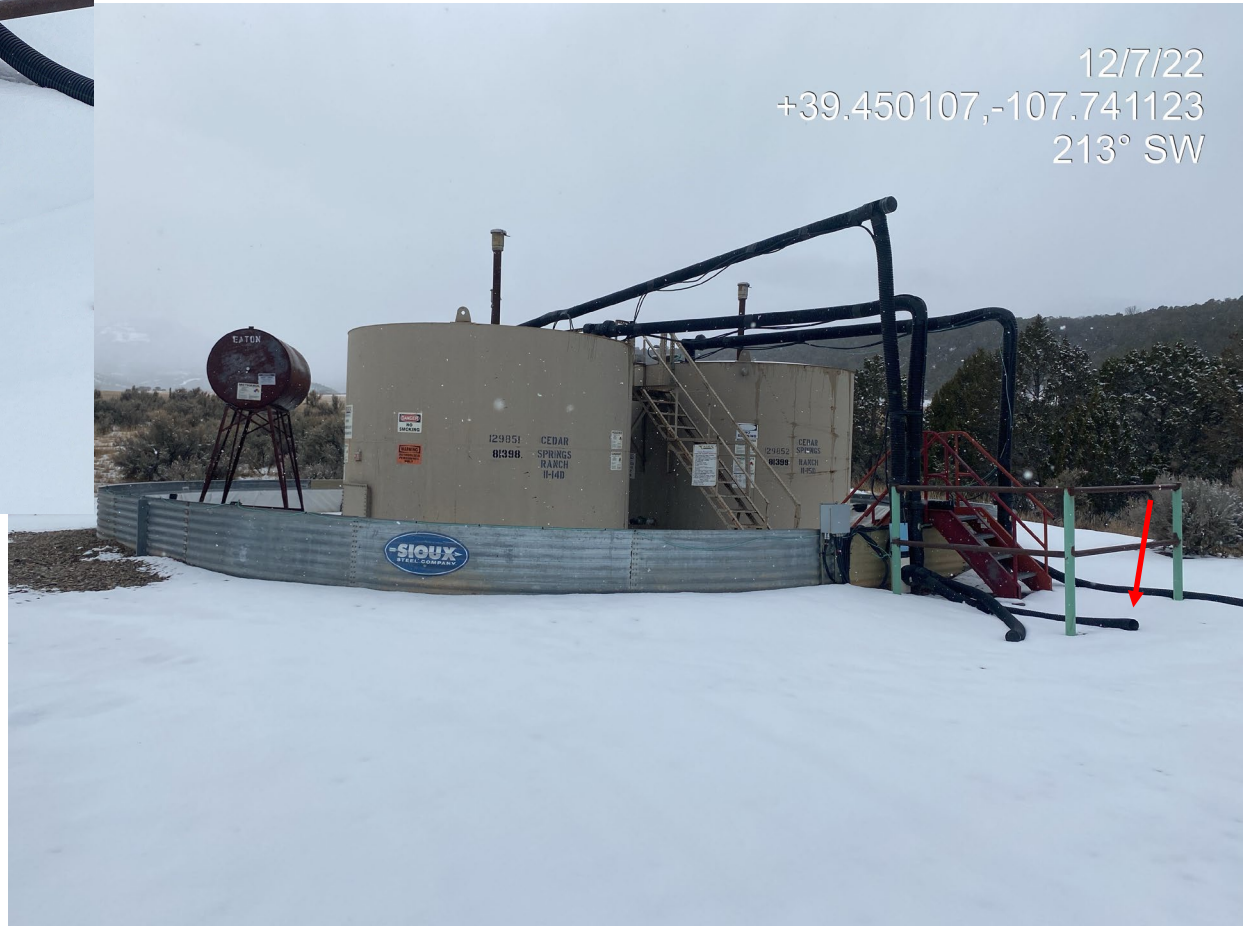
Photo 2. Photo shows production areas. Piping is open ended/uncapped allowing for wildlife access.
