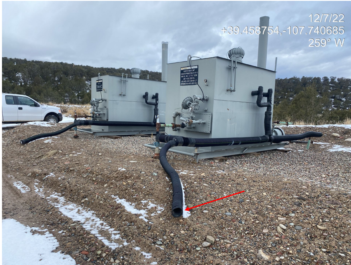
Photo 2. Photo shows production areas. Separator piping is open ended/uncapped, allowing for wildlife access.
