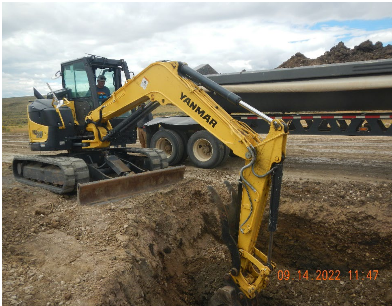
Photo #1 Approximately 130 tons of soil was removed and hauled for disposal as E&P waste.
