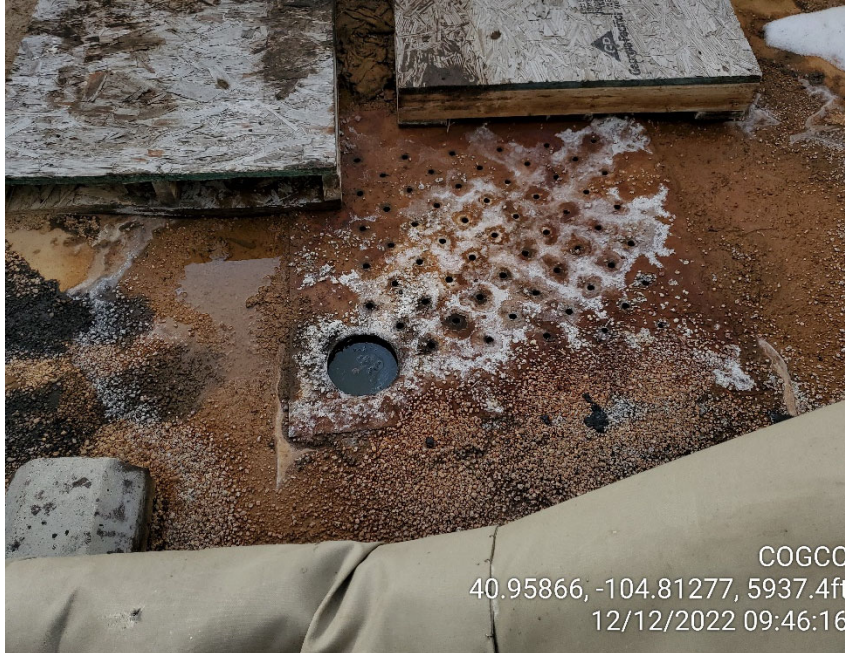
Photo 1 Sump in southwest corner of lined secondary containment at tank battery.
