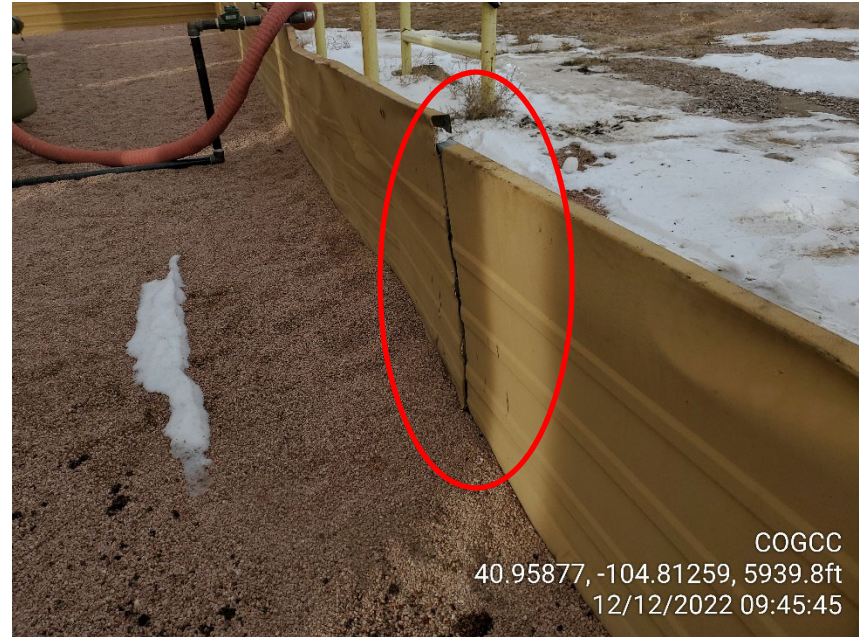
Photo 4 Joint in containment wall with cap in liner.
