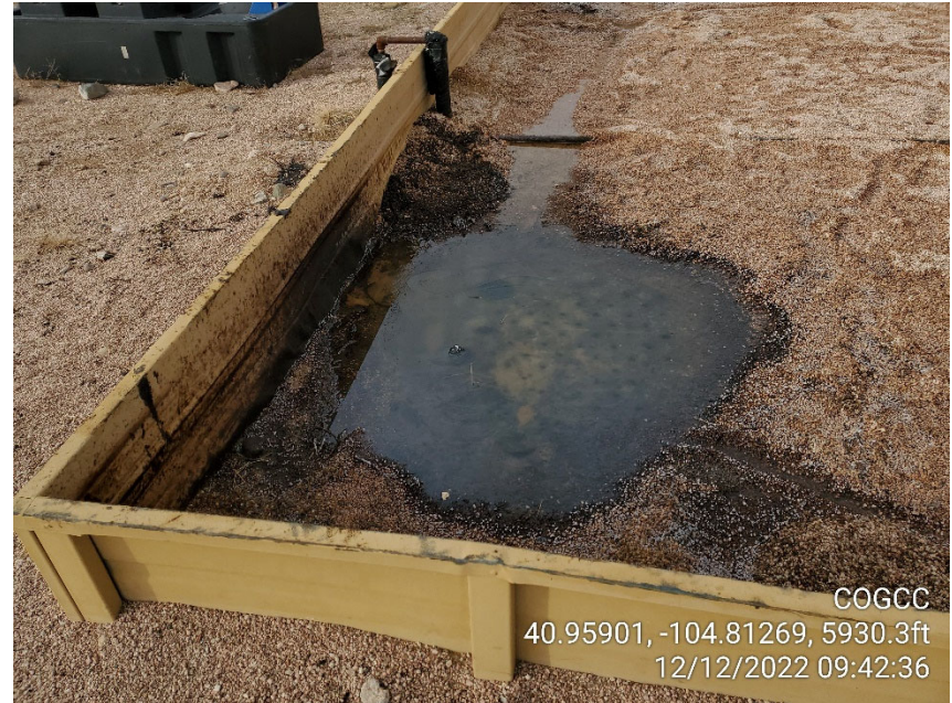
Photo 2 Sump in southeast corner of secondary containment at separator.
