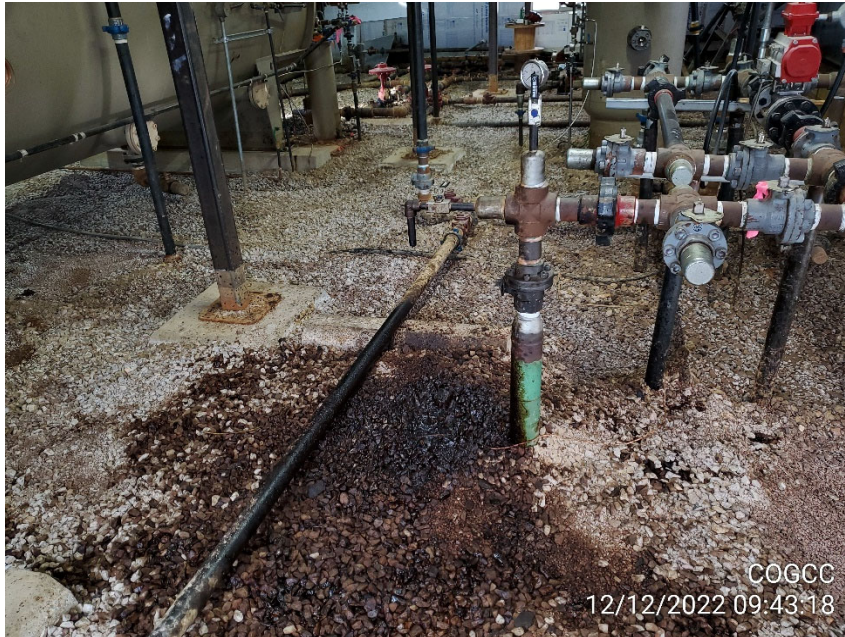
Photo 3 Oily waste from blowdown of production lines.
