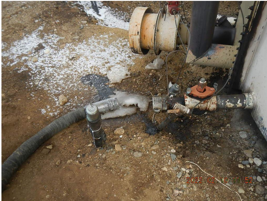
Photo 7. 500 bbl crude Tank #10N79K23 staining on the ground at load valve and coupling. From February 10, 2022 Inspection (Doc #402958096).
