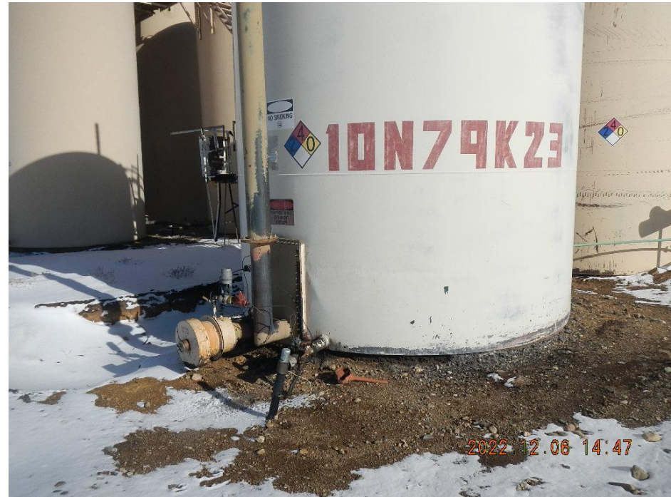
Photo 8. 500 bbl crude Tank #10N79K23 staining on the ground at load valve and coupling appears to have been removed. From December 6, 2022 Inspection (Doc #6900900228).
