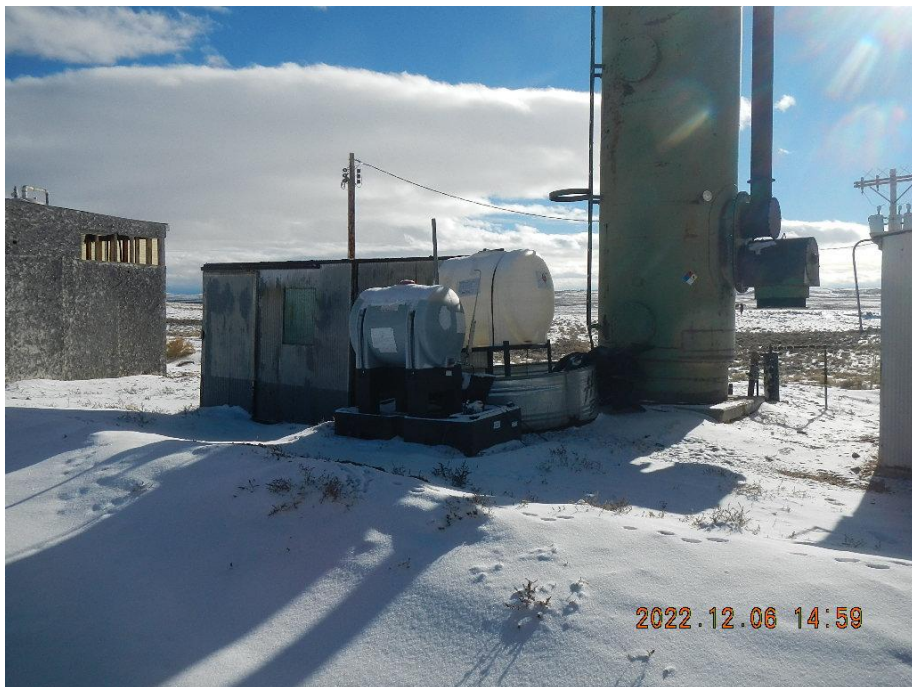
Photo 5. Chemical tote “Paraffin Solvent” in lined secondary containment. Note: The secondary containment has an approximate 6’ to 8’ hole in it. This has been observed in previous inspections.
