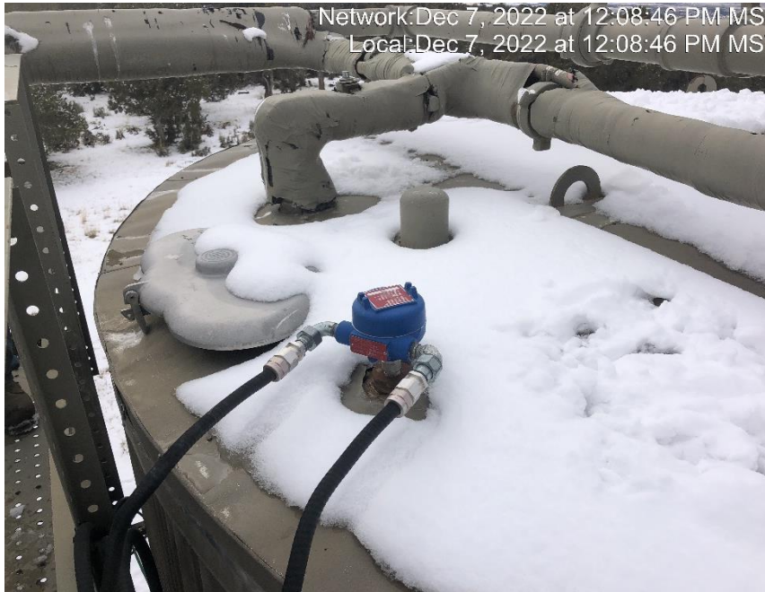
Photo #8614 Multiple gauge hatches leaking refer to OGIS.
