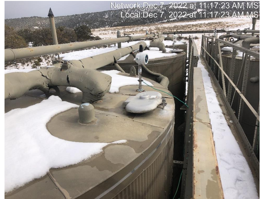
Photo #8581 Multiple leaking Gauge hatches refer to OGIS
