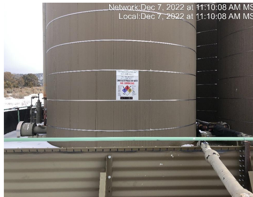
Photo #8579 Tank label weathered and not legible.
