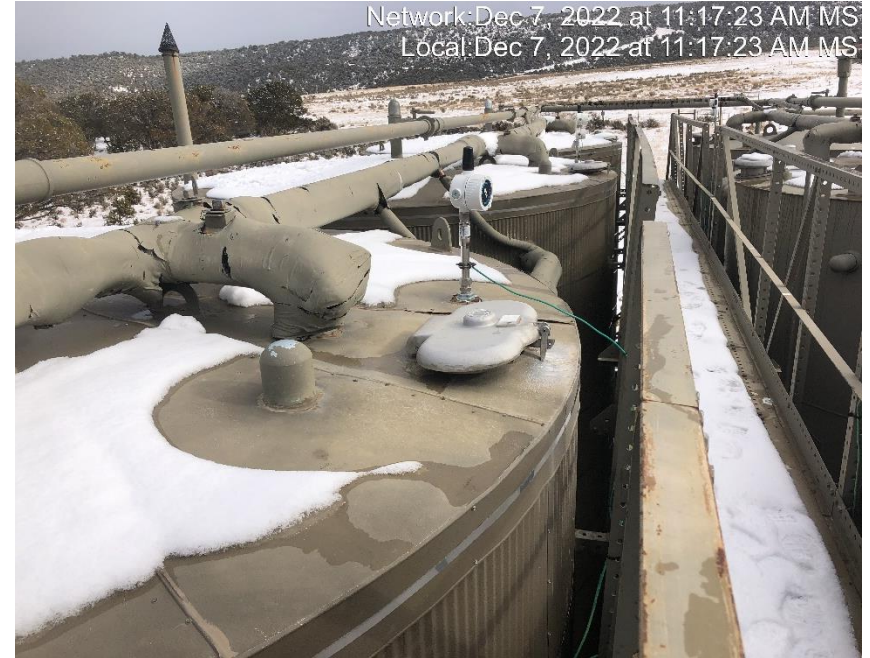
Photo #8570 Multiple thief hatches leaking refer to OGIS.
