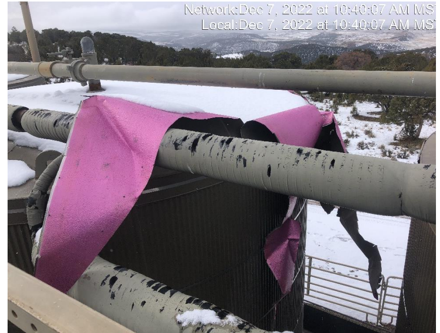
Photo #8570 Tank insulation needs repaired.
