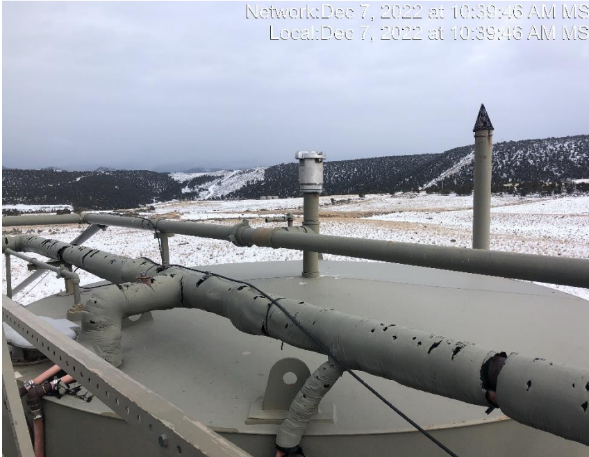
Photo #8569 PRV leaking Referto OGIS.
