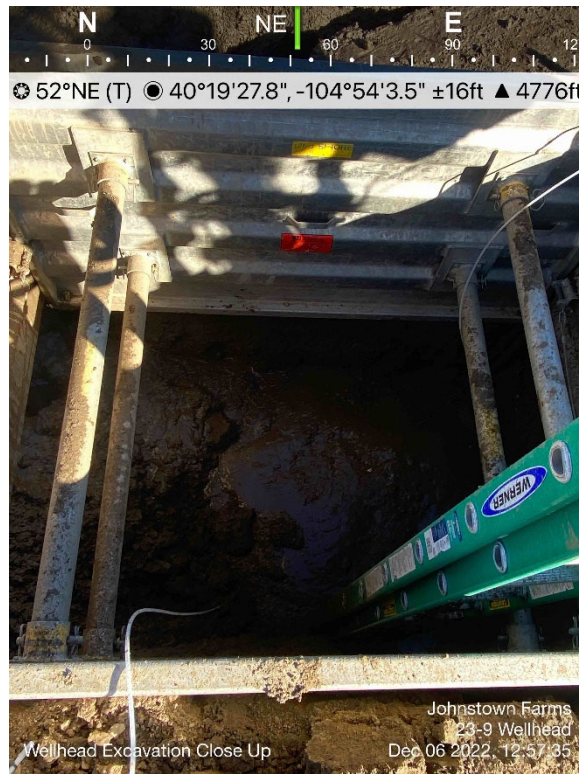
Wellhead Excavation Close Up (Hydrovac Water in base of excavation)
