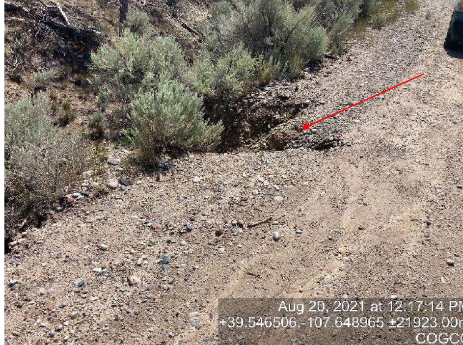
Photo 5. Photo shows access road erosion from the 12/7/22 inspection (left) and previous 8/20/21 inspection (right).
