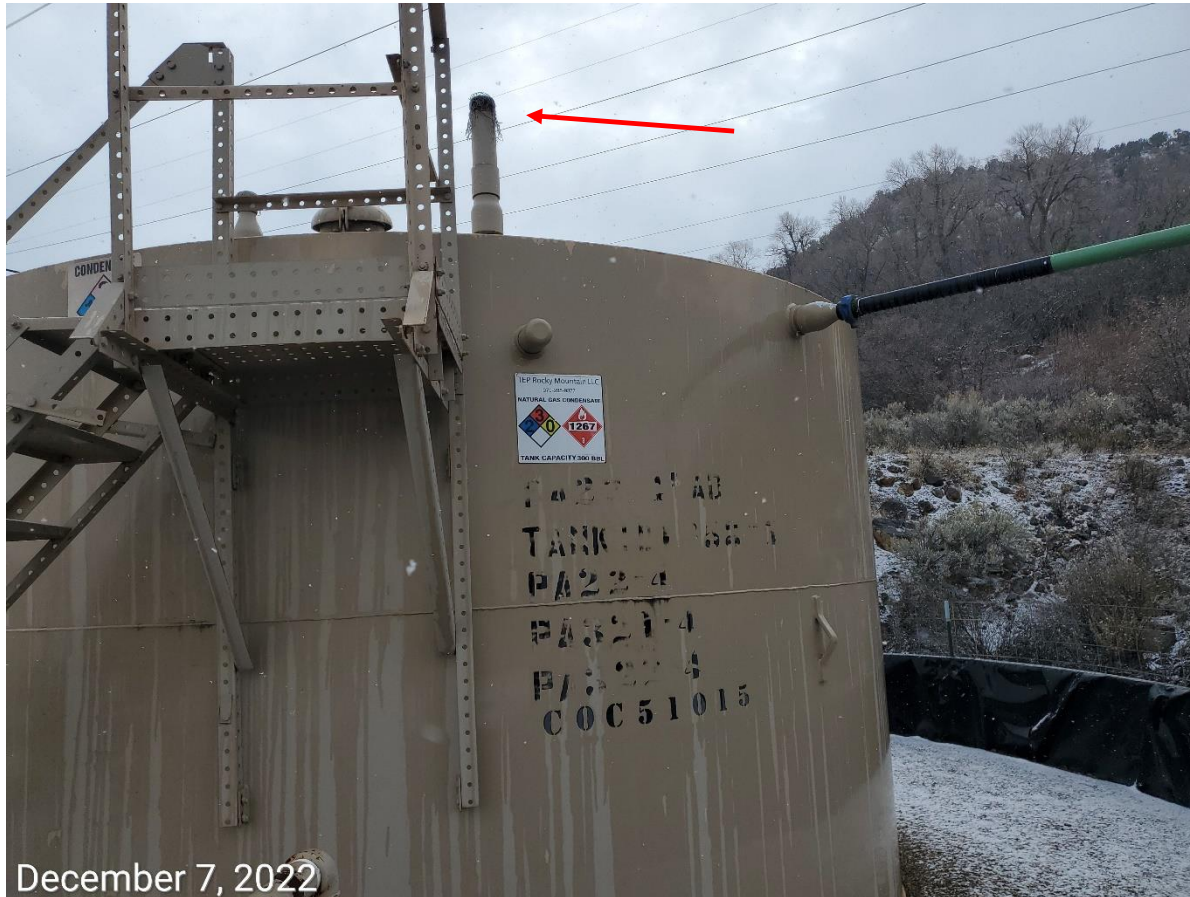
Photo 3: Photo shows open valve at the condensate tank has been covered with wire netting.
