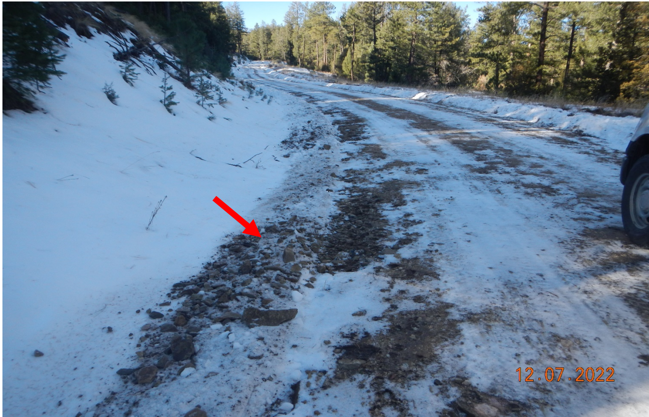
Photo 4. Facing west along the access road. The snow has been recently graded off the road. There erosion issues previously observed are now obscured by snow cover, Grading of the road has pushed some of the rock dams up shown at red arrow.
