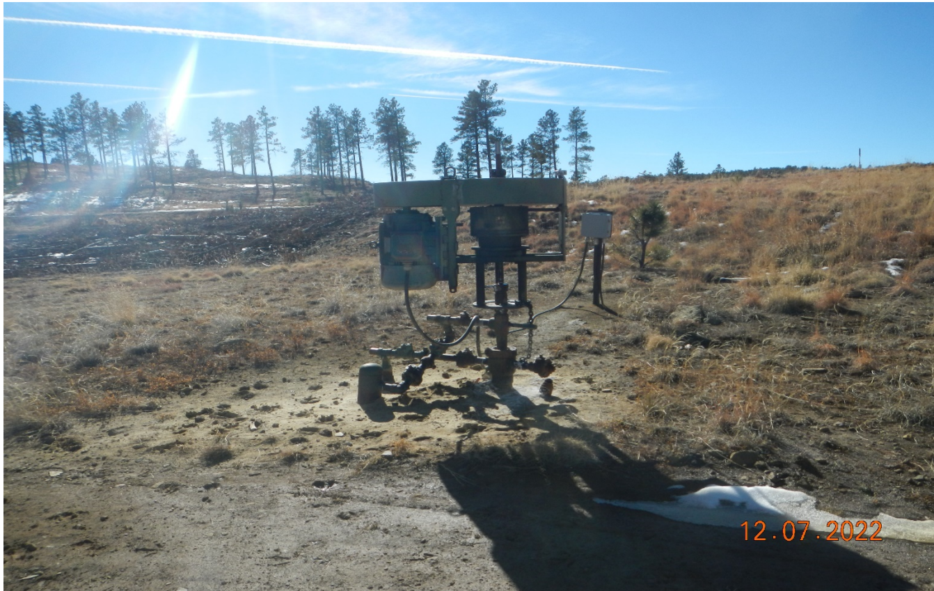
Photo 3. Facing toward the wellhead.
