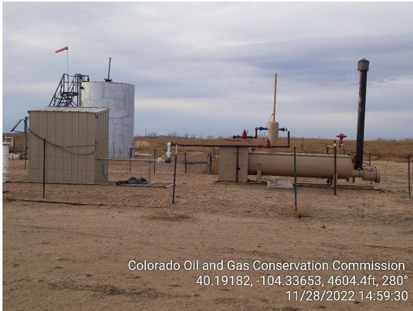
Photo 3 – Separator and Gas Meter
