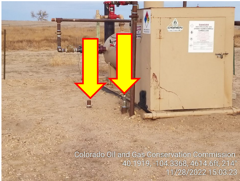
Photo 7 – Unmarked Risers at Separator
