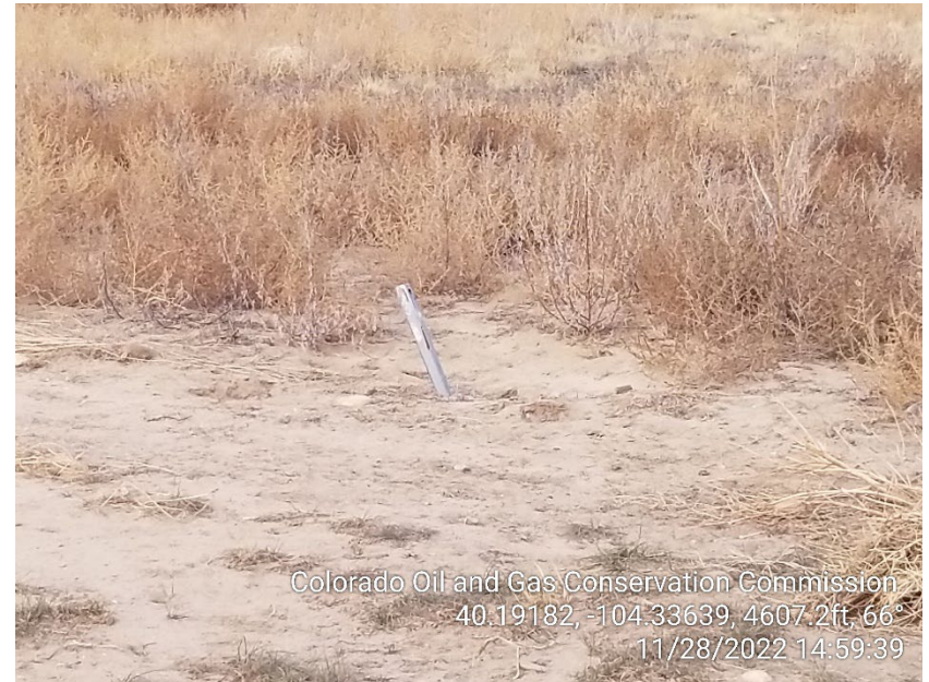
Photo 4 – NE Deadman Anchor NOT Marked
