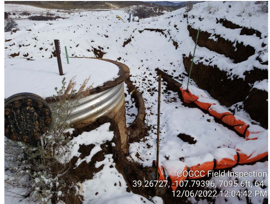
Photo #4 – View inside of excavation. Hydrocarbon odors were observed in this area during inspection.
