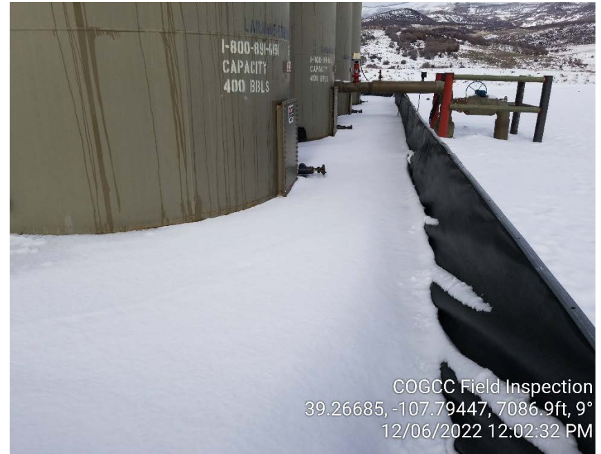
Photo #8 - View into east side of tank battery secondary containment.
