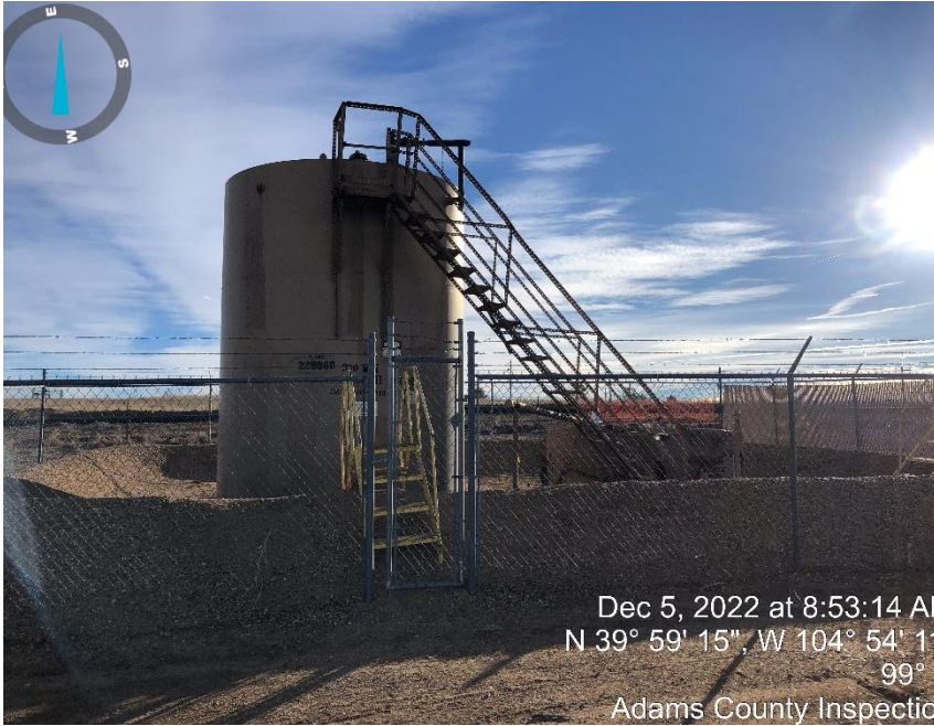
Photo# 1 Crude tank & P/R water tank.
