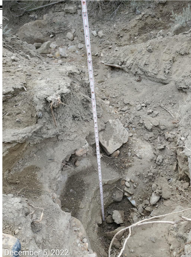
Photo 4: Continued from photo 3. Erosion observed at access road ~3.5 to 4 feet deep.
