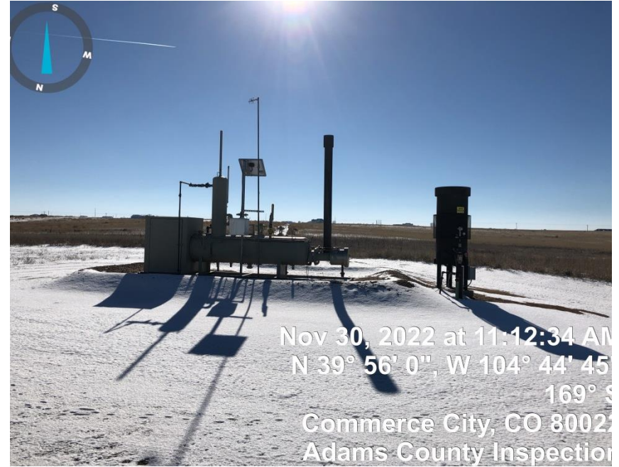
Photo#2 Separator/ECD/Automation RTU
